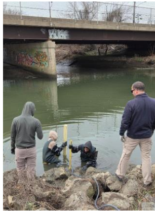
84 th St. Bridge
