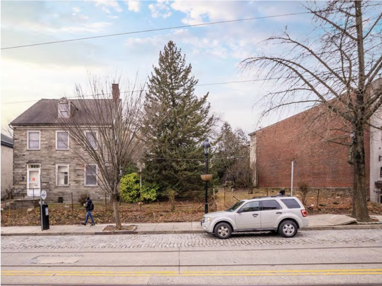
Figure 2: View of front of 8226 Germantown Ave from Germantown Ave (from application):
