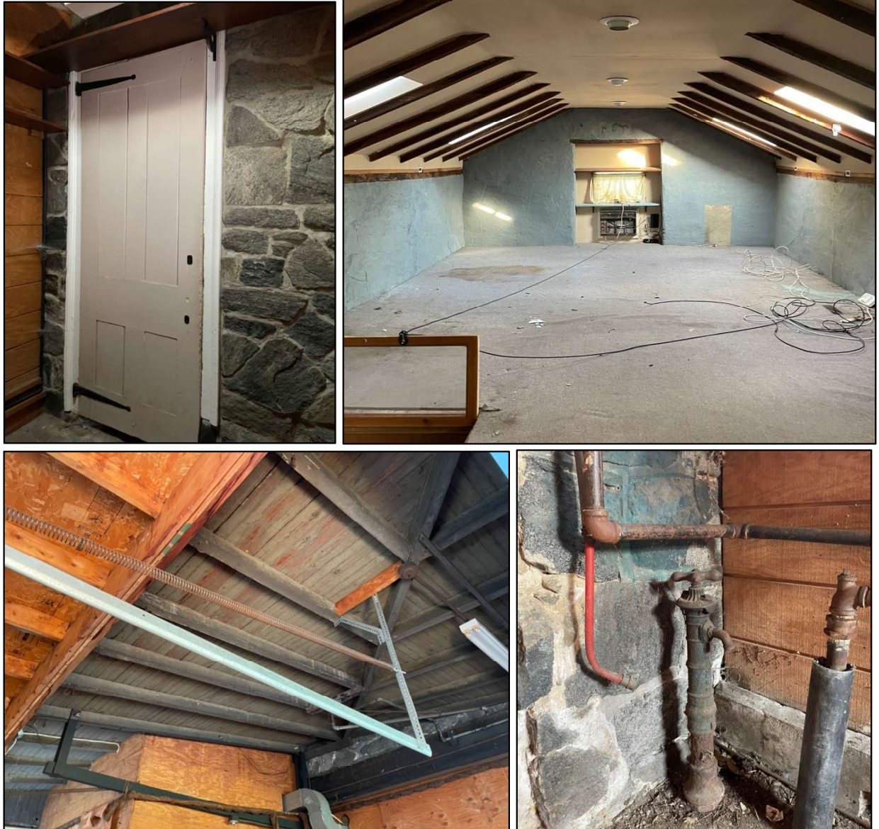
Fig. 42, top left. The door to the Carriage House's south wall, now enclosed in the Garage dating from ca.1906-1911. Fig. 43, top right. The loft in the Carriage House. Photos: SoLo Germantown. Fig. 44, bottom left. A view of the underside of the original south porch overhang at the Carriage House. It had later been expanded into a garage. Fig. 45, bottom right. An older water spigot at a once exterior location, now enclosed in the Garage.
