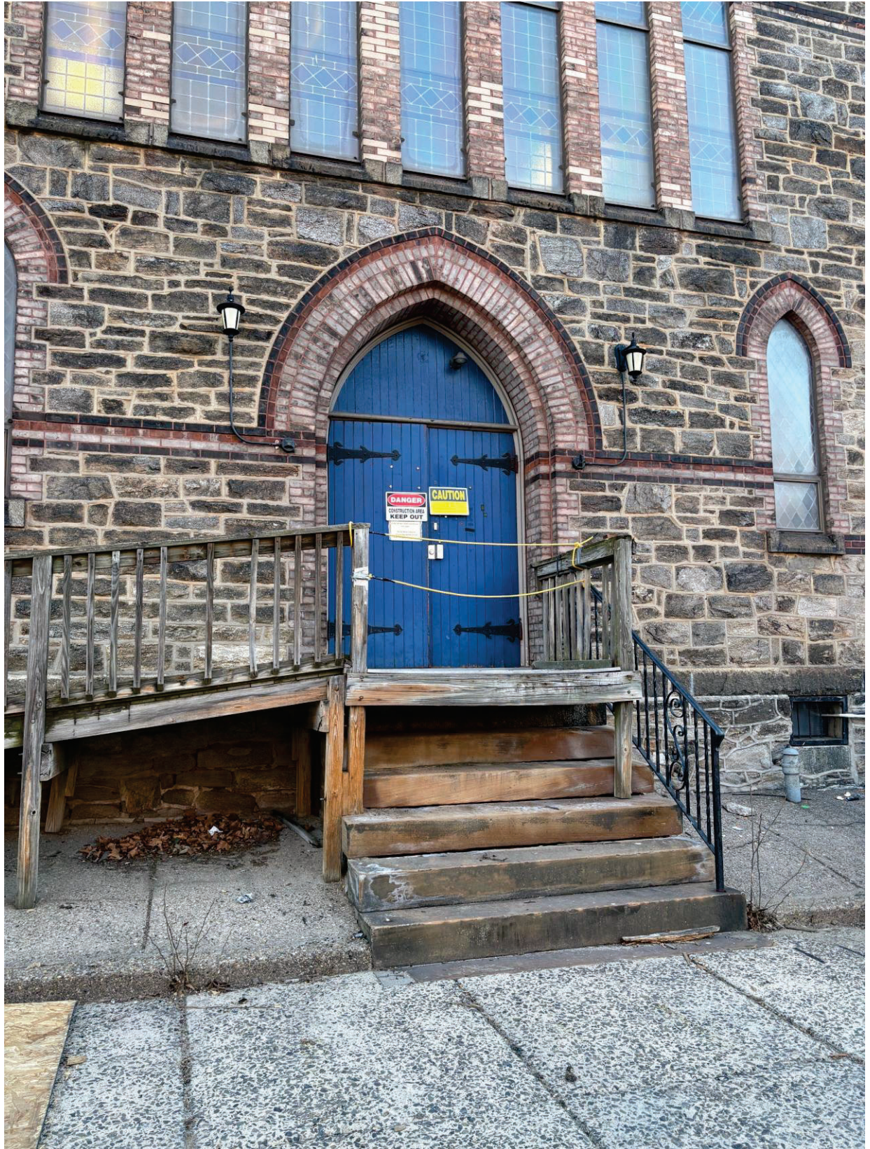
Image 3: Current entrance on west elevation. The existing wood ramp is proposed for removal. The door, stairs and railing will be rehabilitated.
