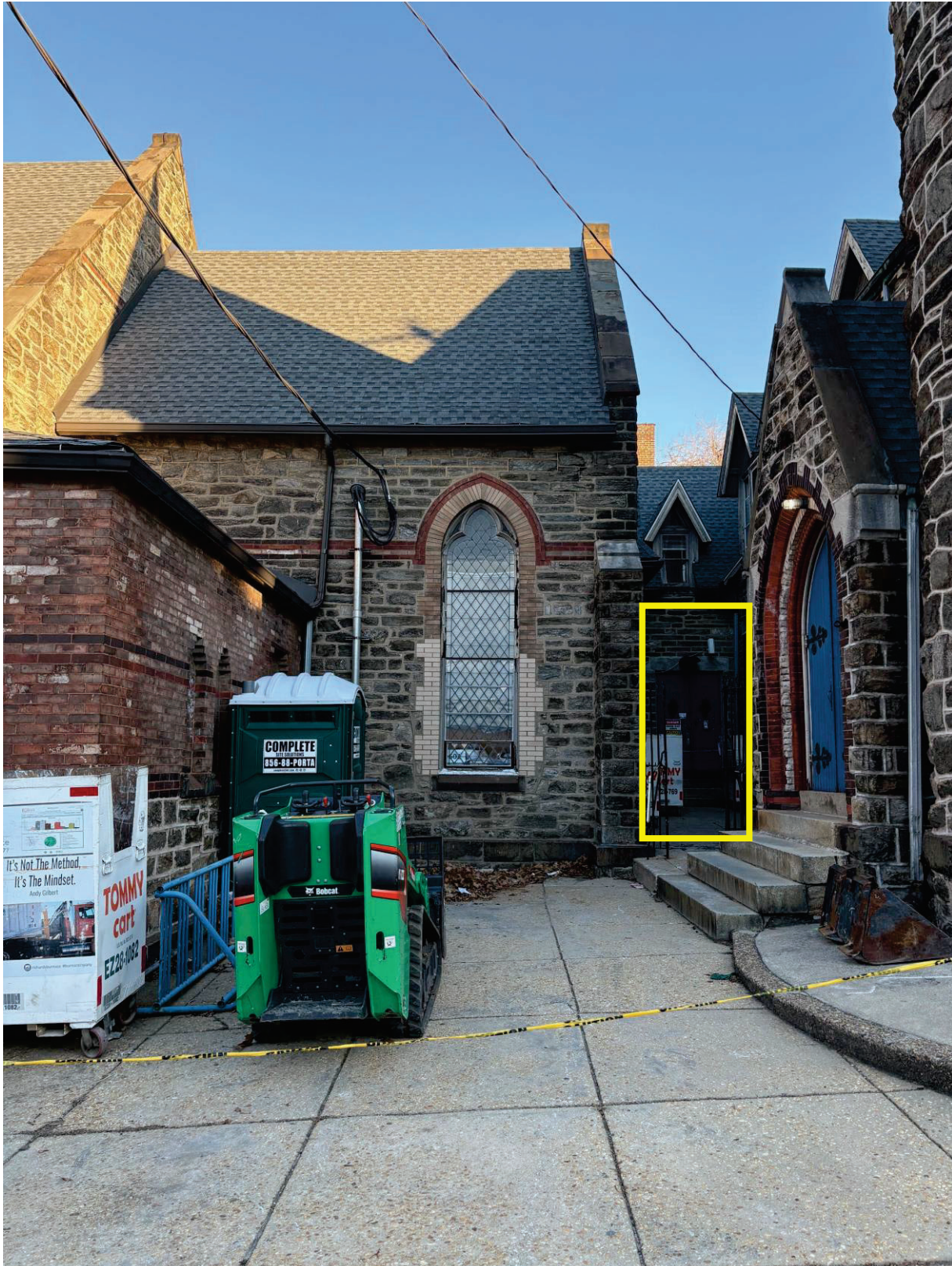
Image 2: Close up view of area of south elevation. A new entrance courtyard with gate, signage, paving, side door, and entrance vestibule is proposed for this exterior space. The location of the new vestibule is indicated in yellow.
