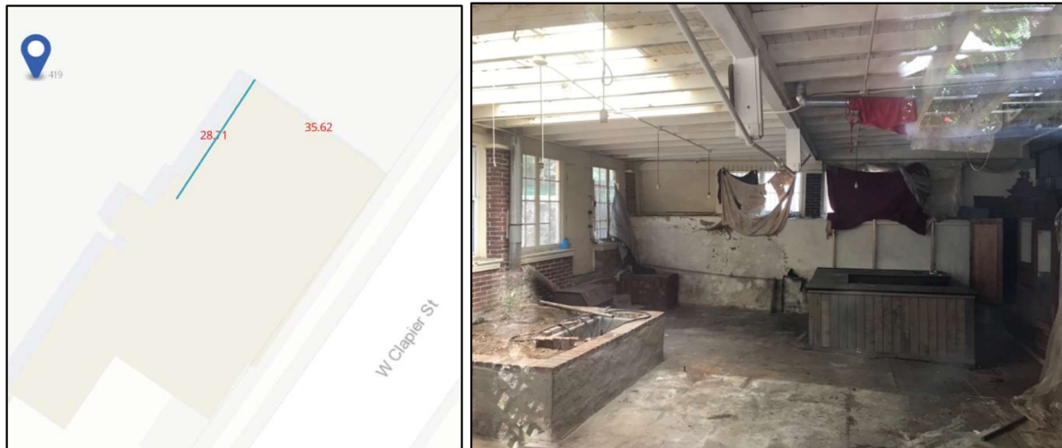
Fig. 56, left. Dimensions of the existing Greenhouse from Atlas match those given in the 1905 announcement of its construction (35' x 28'). Fig. 57, right. The Greenhouse as it appeared in 2025 with a piped, concrete basin under roof glazing. Photo: SoLo Germantown.
