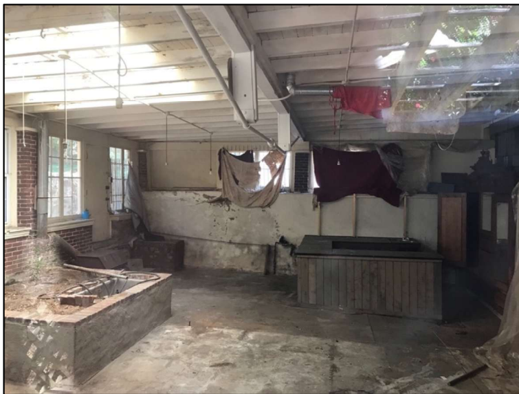
Fig. 25. The interior of the Greenhouse from the garden-facing windows. There is glazing in the roof at northern side of the building and below it what seems to be a piped concrete basin that allowed for goldfish or permanent plantings. The floors are exposed concrete and there is no insulation at the ceiling rafters. The east side (opposite) shows the windows on each far end boarded up by plywood (and faced at the exterior by shingles). There is a parge coat on the interior side of the east perimeter schist wall with a more structured sill below the windows. Date: August 11, 2025.
