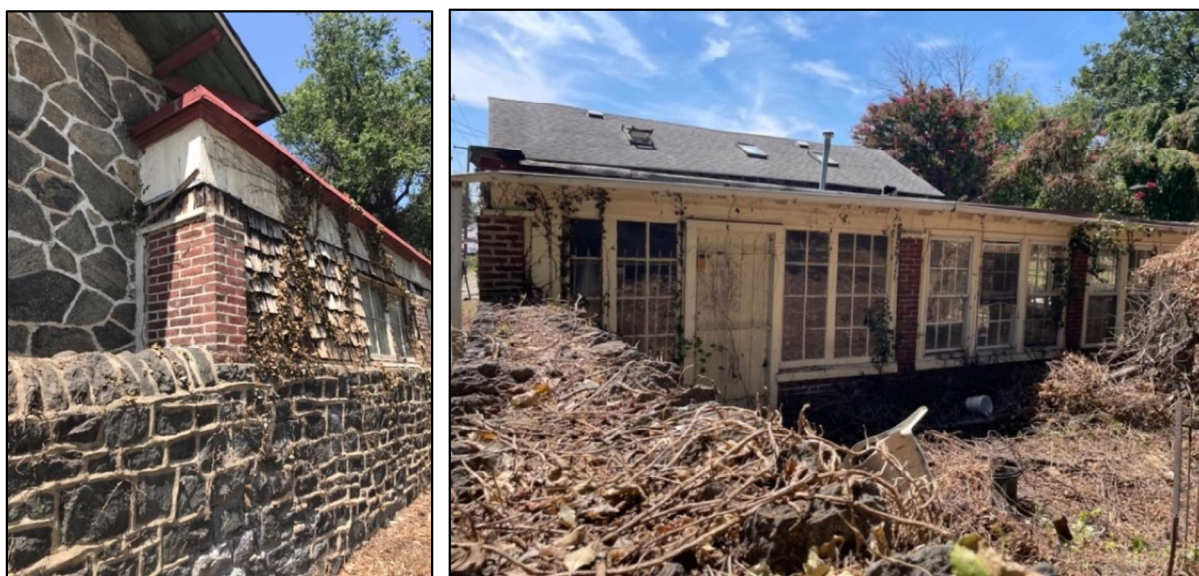
Fig. 22, left. The north walls of the Carriage House and the Greenhouse intersect with each other, and the solarium wall rises from the perimeter schist wall. Fig. 23, right. The north wall of the solarium showing the extensive fenestration along this elevation with low sills in the brick wall and a couple of brick pilasters breaking up the window openings. An access door is located closer to the east side of this elevation. The roof field of the stone building beyond can be seen with skylights. Far left foreground is the top of the perimeter schist wall. Photos: August 9, 2025.
