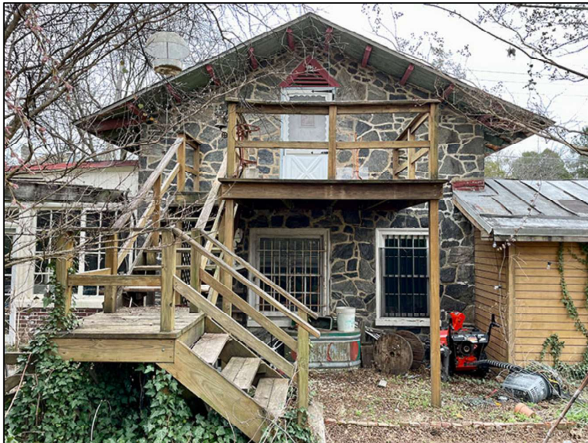
Fig. 21. The west elevation of the stone building facing the garden and showing the connections to the garage to the south (right) and to the solarium to the north (left). There are two window openings at the lower level which do not appear to have been altered from door structures; each contains wood frames and divided lite windows. Date: March 28, 2025.
