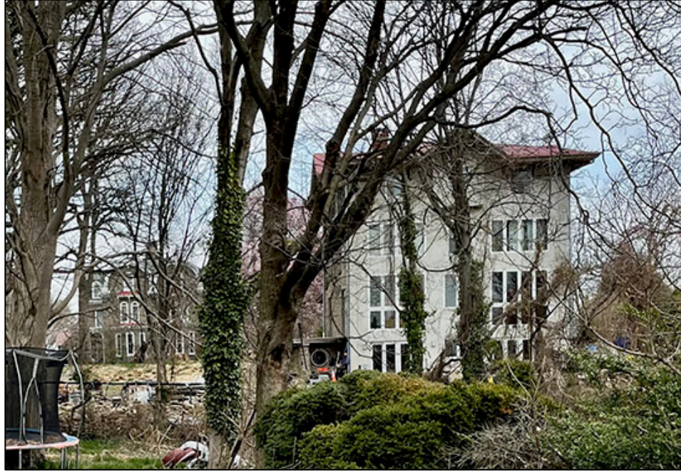
Fig. 12. Photo of the south (rear) elevation with its non-historic stucco coat and windows. To the left is the garden side porch slab with its cellar-level round window. Photo: SoLo Germantown, March 2025.
