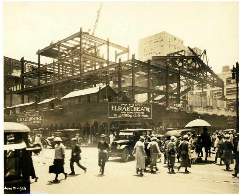
Figure 22: Photo of the Earle Theatre (then called the Elrae) under construction shows the steel skeleton under the masonry façades. Photo from the Glazer Theater Collection.
