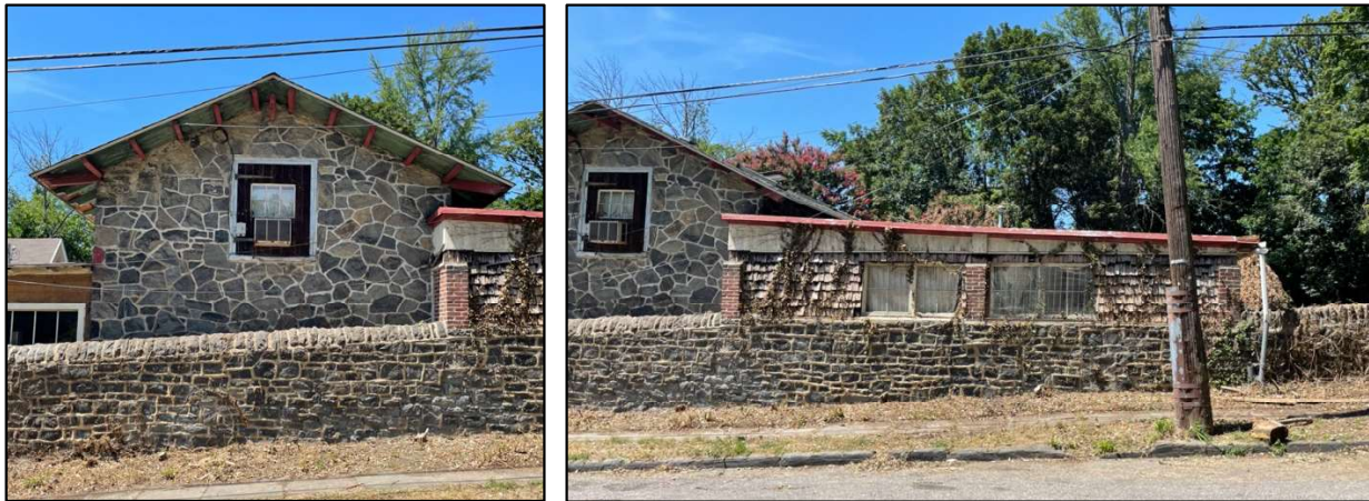
Fig. 19, left. The east elevation of the Carriage House between the Garage to the south and the Greenhouse to the north. Fig. 20, right. The east elevation of the Greenhouse to the north of the Carriage House. The shingled panels are not original; they cover window sashes. The base of the east Greenhouse wall is flush with the later perimeter wall on either side. Photos dated August 9, 2025.
