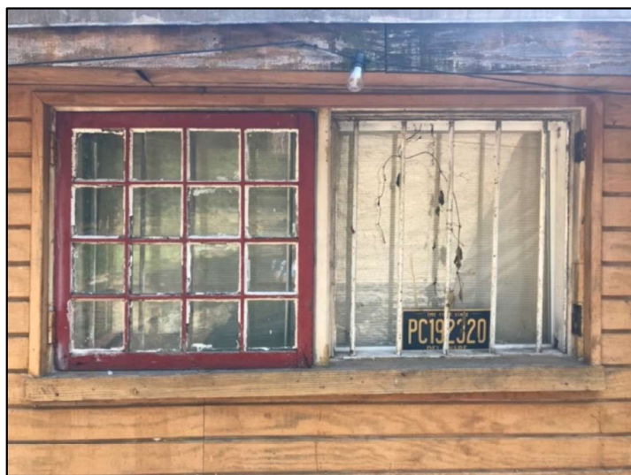
Fig. 15, left. The junction of the north elevation of the Carriage House and the Coachman's Residence. Date: July 27, 2025. Fig. 16, right, the southernmost window opening in the west elevation of the garage's workshop extension showing what may be an original cased wood window with divided lites. Date: August 9, 2025.
