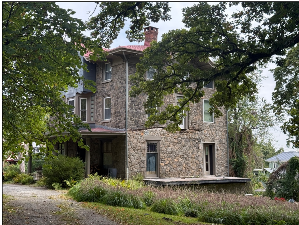
Fig. 13. Photo of the west (side garden) side elevation of the house with its historic porch slab but without a roof structure indicated by the ghosting on the masonry wall. Photo: SoLo Germantown, September 2025.
