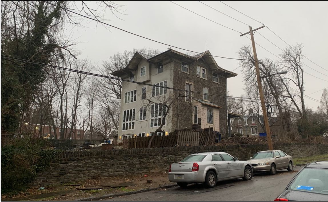
Fig. 11. View of the dwelling from West Clapier Street looking at the south (rear) elevation with a layer of stucco and contemporary windows in the historic, 3-bay configuration. The perimeter schist wall extends from McKean Avenue (right) along the entire Clapier St. frontage. Photo: SoLo Germantown, March 2024.
