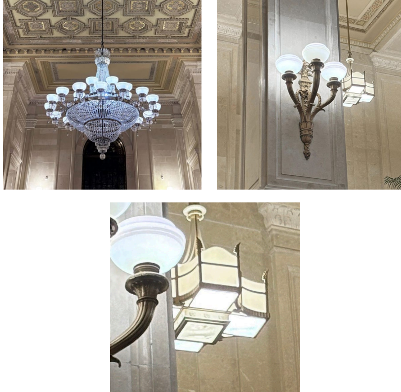
Figure 13: Clockwise from top left: The crystal chandelier within the Main Banking Room (1 fixture), the bronze sconces on the four walls of the space (12 fixtures total), and the hanging pendant fixtures on the mezzanine (10 fixtures total).
