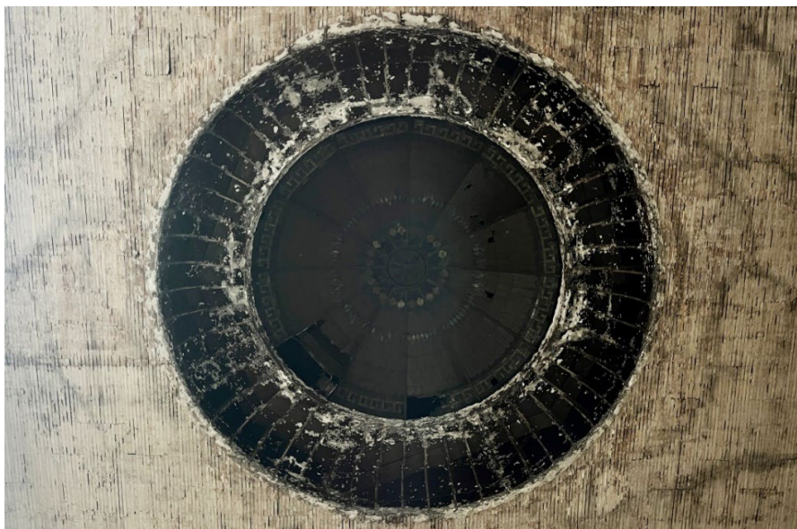
Photo 13: Leaded-glass dome at the center of the banking hall ceiling. The glasswork is largely intact, but the plaster finish on the cove below it (the wide ring surrounding the glass) is largely missing.
