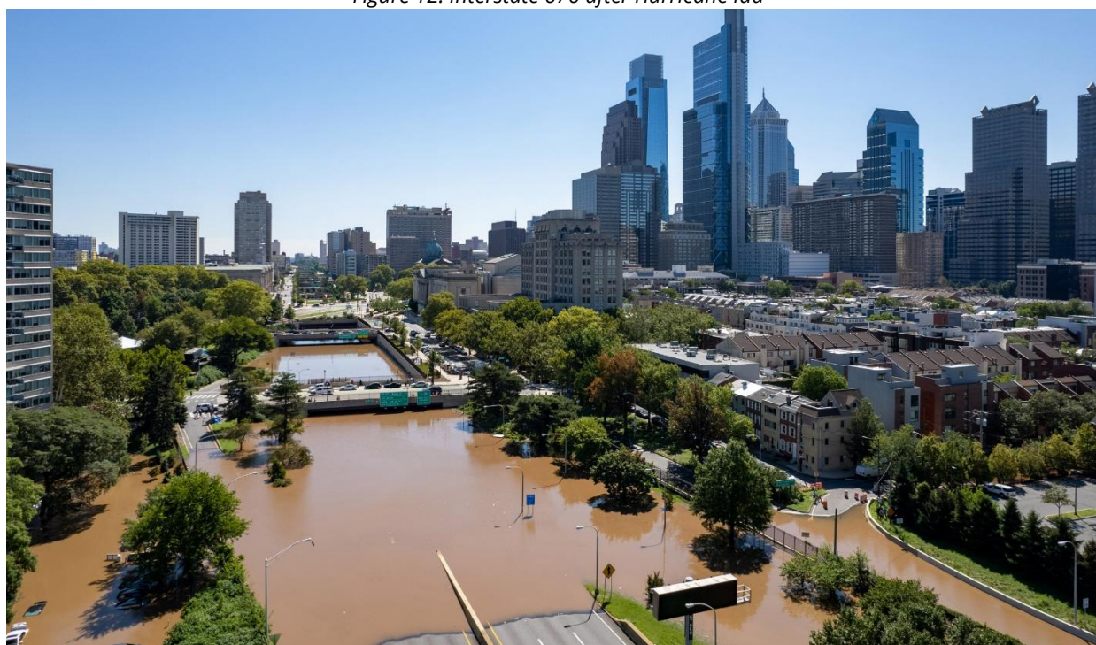
Figure 12: Interstate 676 after Hurricane Ida
