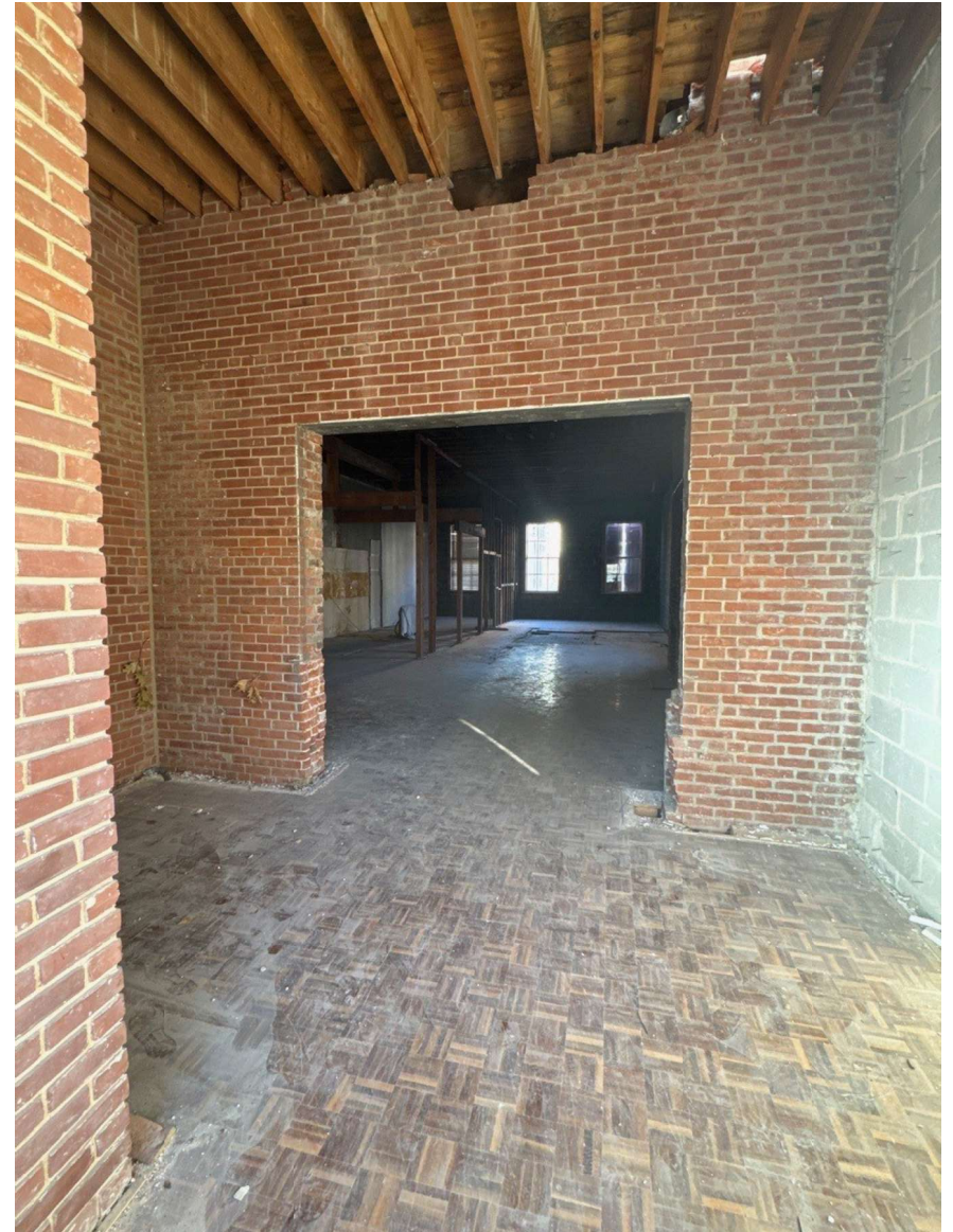
SECOND FLOOR EXISTING REAR OPENING LOOKING WEST
