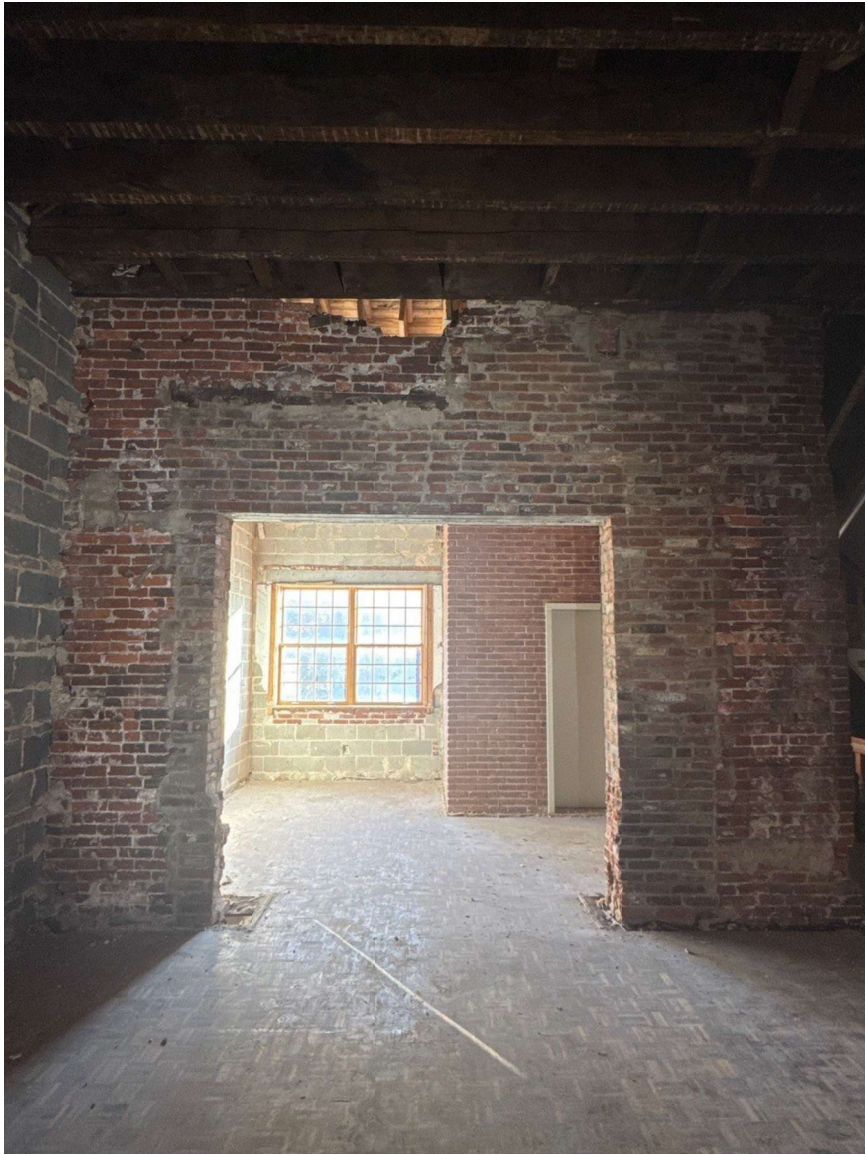
SECOND FLOOR EXISTING REAR OPENING LOOKING EAST
