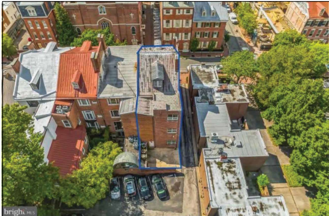
REAR OF PROPERTY LOOKING TOWARD 4TH STREET
