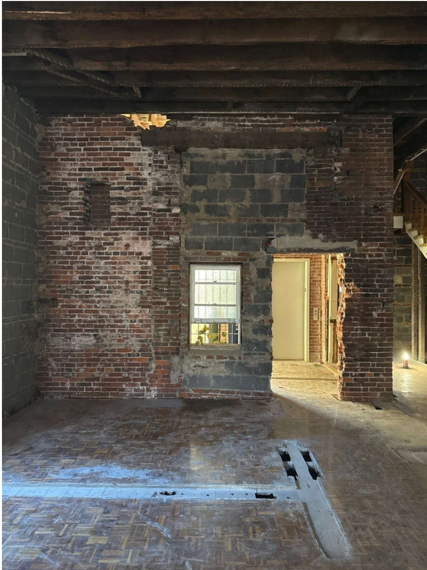
FIRST FLOOR EXISTING REAR OPENING LOOKING EAST
