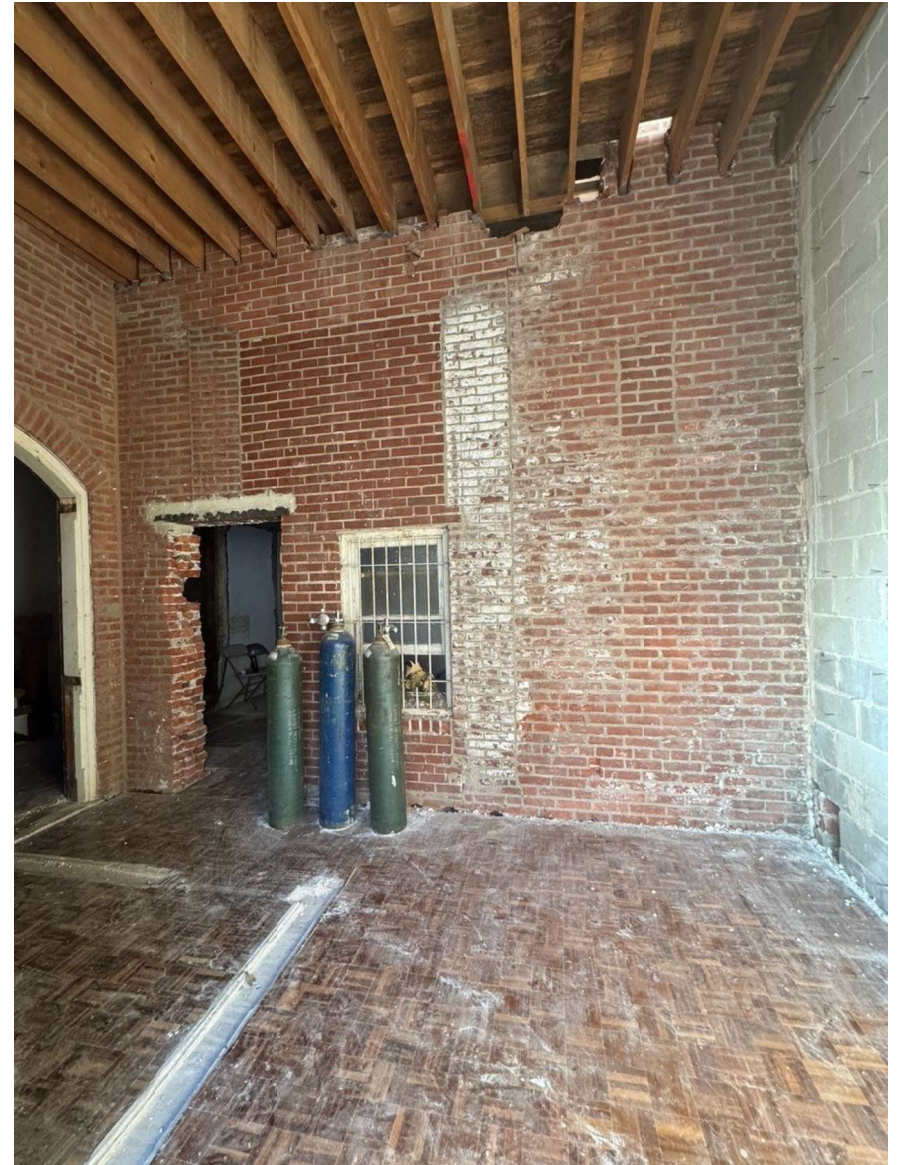
FIRST FLOOR EXISTING REAR OPENING LOOKING WEST
