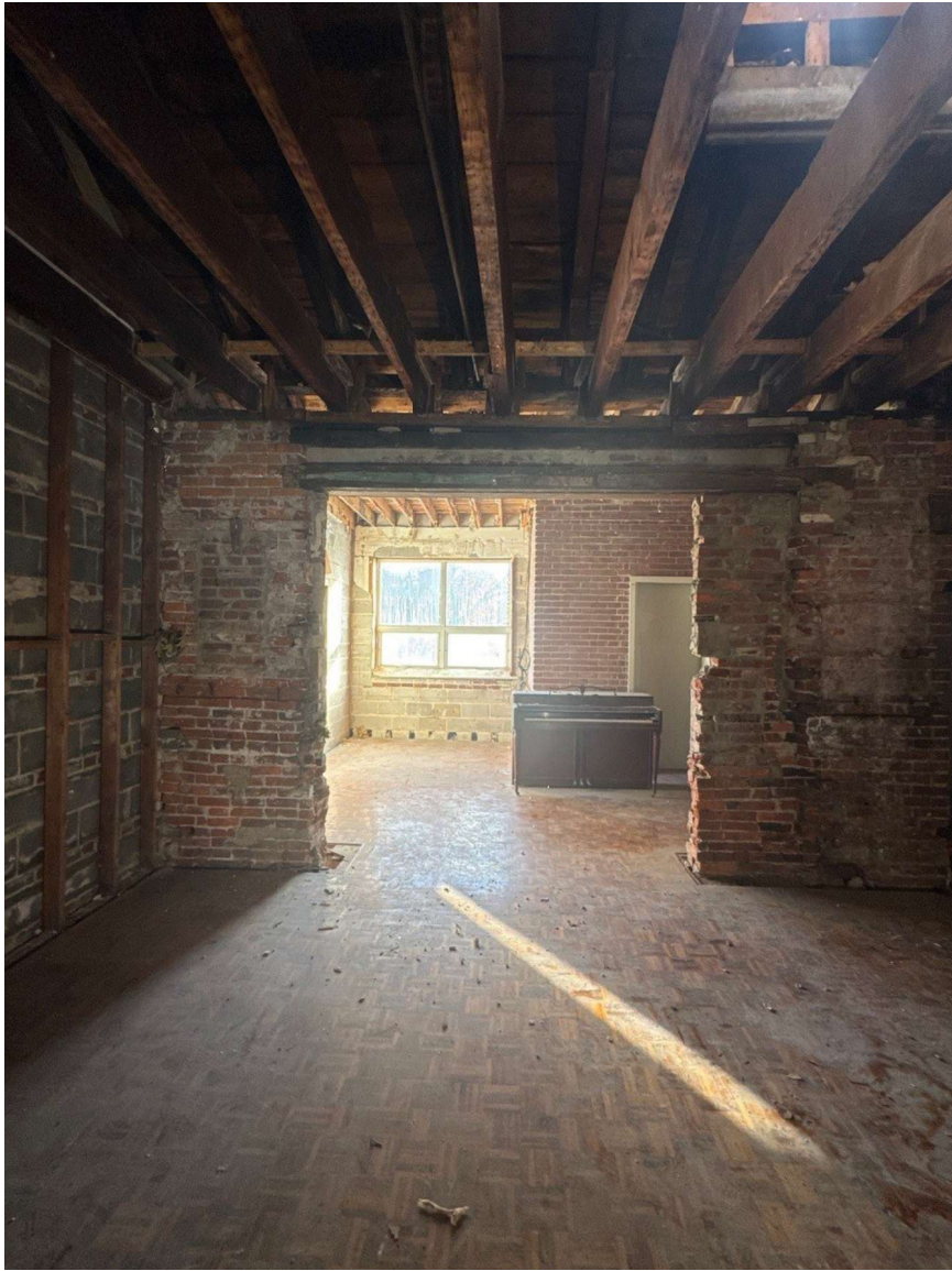
THIRD FLOOR EXISTING REAR OPENING LOOKING EAST
