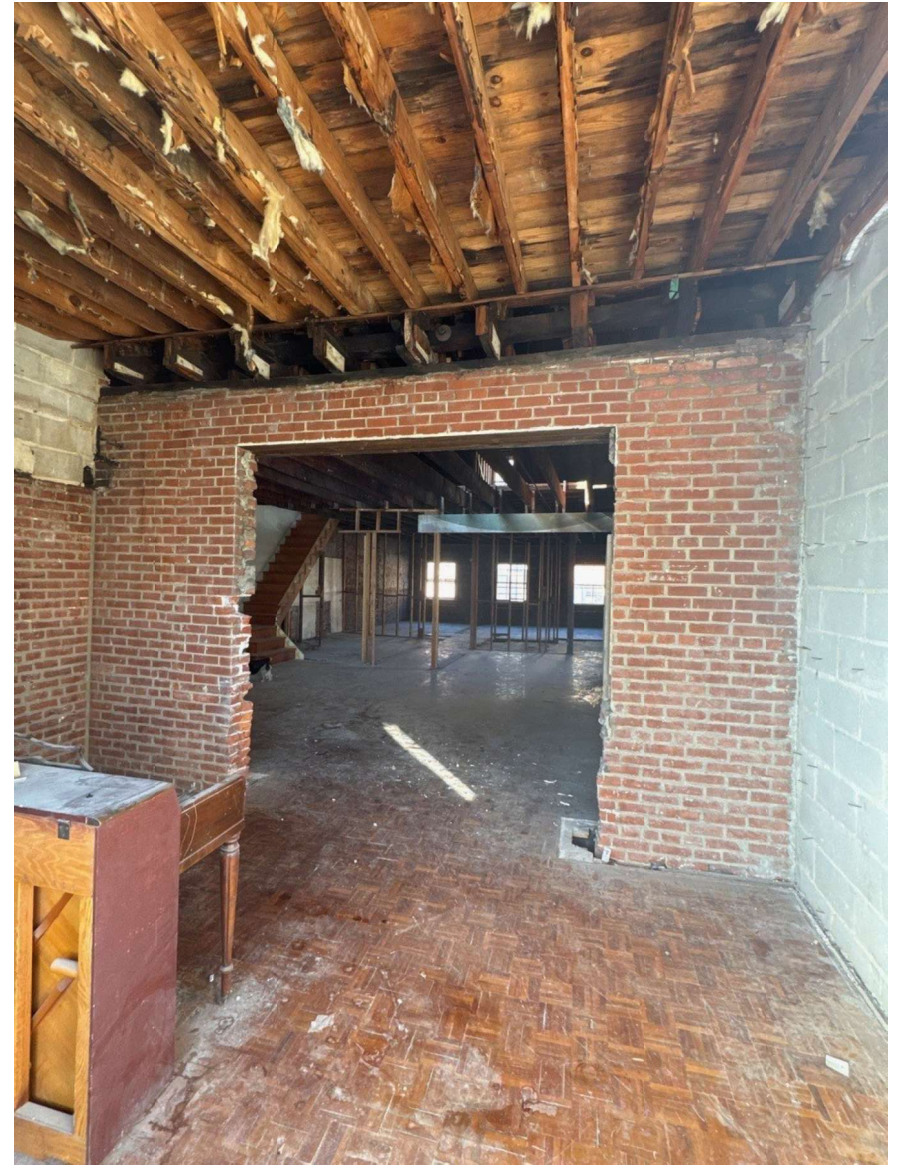
THIRD FLOOR EXISTING REAR OPENING LOOKING WEST
