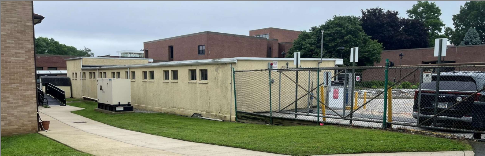
East and North Facades
