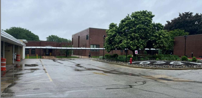
Garage, Bus Drop-Off Area, and East Facade
