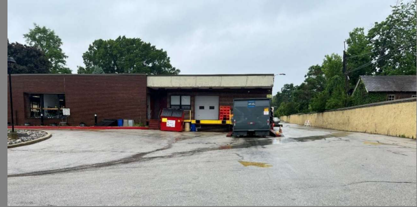
East Facade, Loading Dock and Trash Compactor
