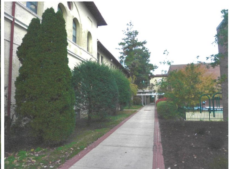
Side and bridge addition
