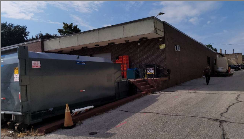
North Facade and Trash Compactor
