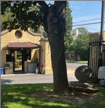
Northeast Vehicular Gate
