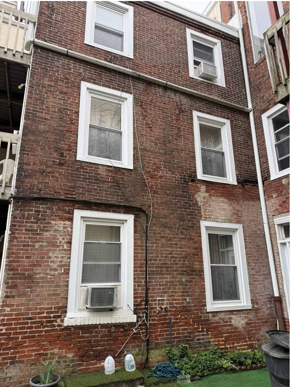
1907 GREEN ST - REAR SIDE VIEW
