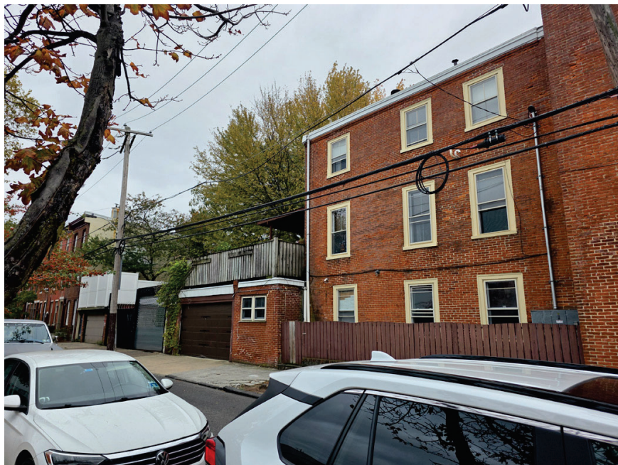
View of North St across from site
