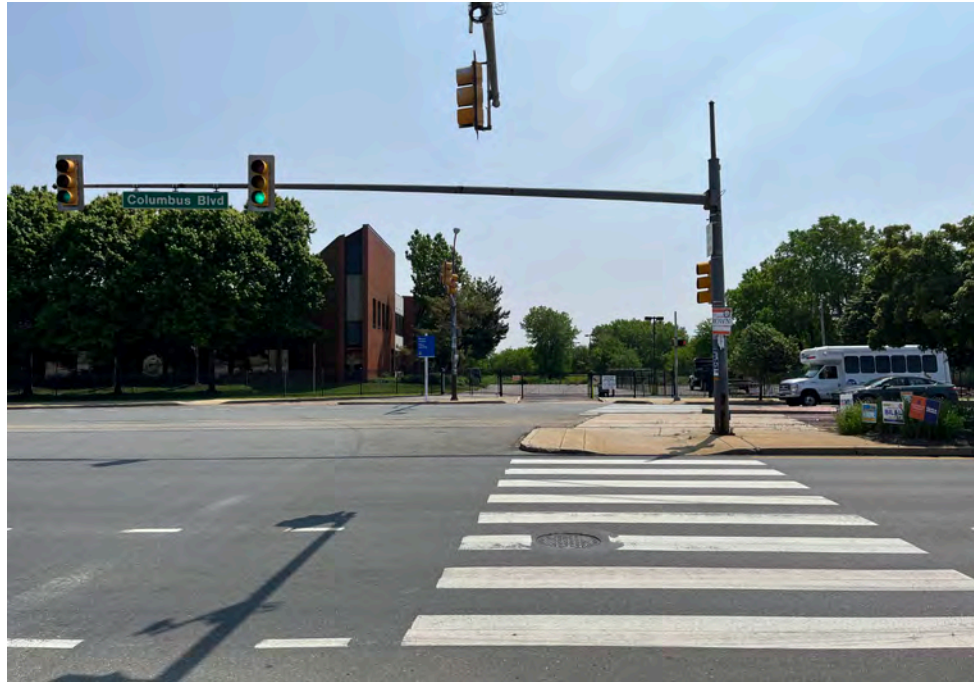
1 I-95 RAMP LOOKING EAST
