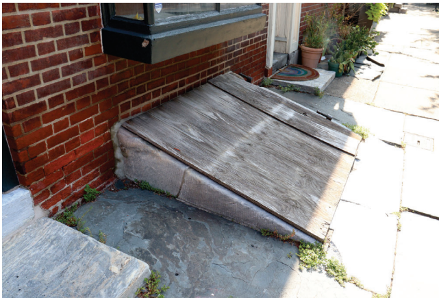
Areaway damage to be repaired, and a new hatch will be added.
