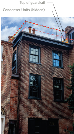
Figure 3: On Camac St, Looking ESE October 2025
