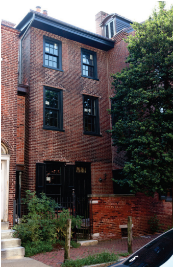
Figure 4: West Elevation, taken from Camac Street July 2025
