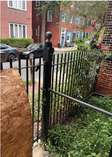
Figure 3: View of metal fence and rail
