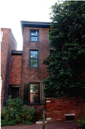
Figure 5: West Elevation taken from Camac Street July 2025
