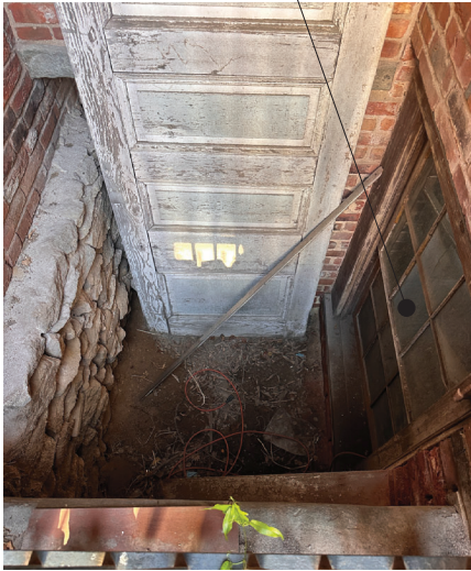
Figure 5: View into well
