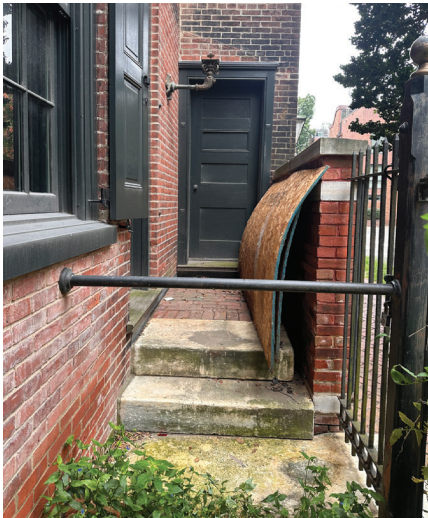
Figure 2: View of side yard looking south
