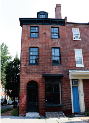
Figure 1: South facade, taken from Pine Street July 2025
