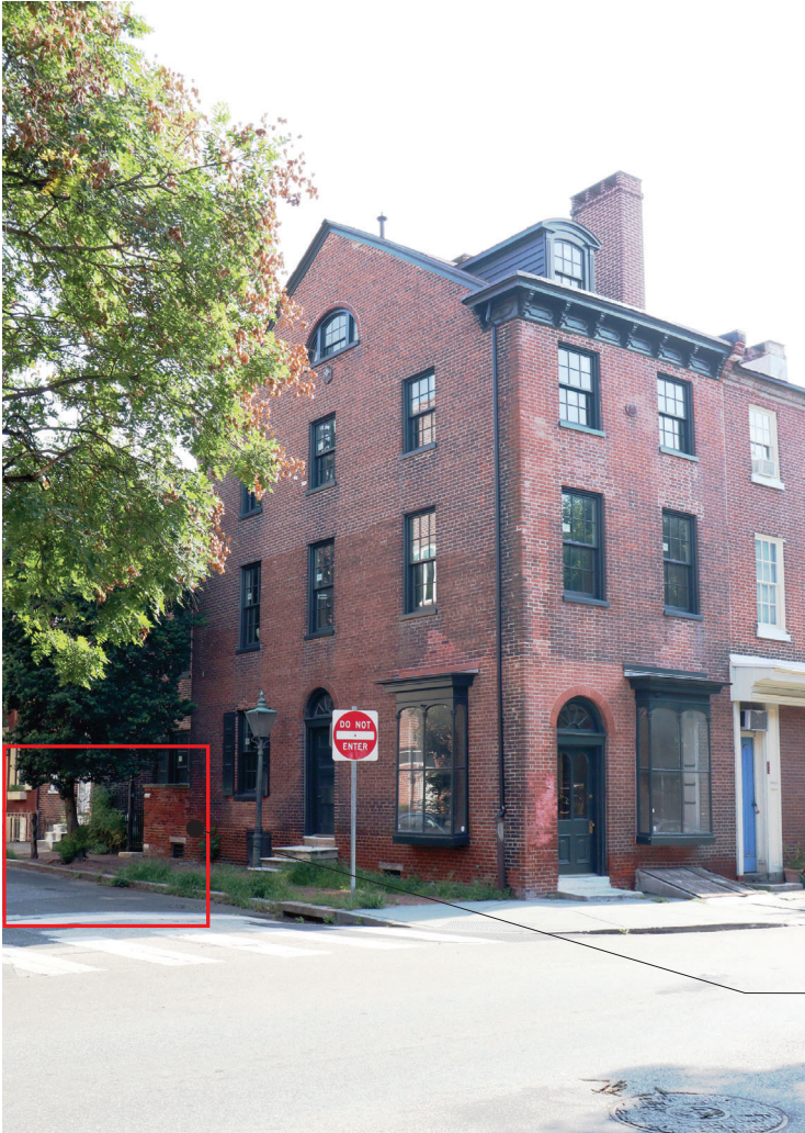
Figure 3: South and West Elevations looking at the intersection of Pine Street and Camac Street, ca. 2025
