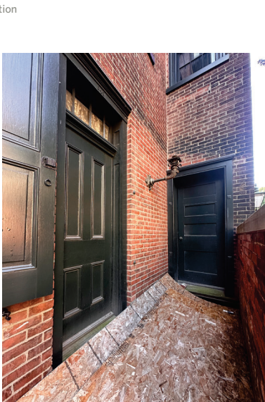
Figure 2: Existing side yard entry doors
