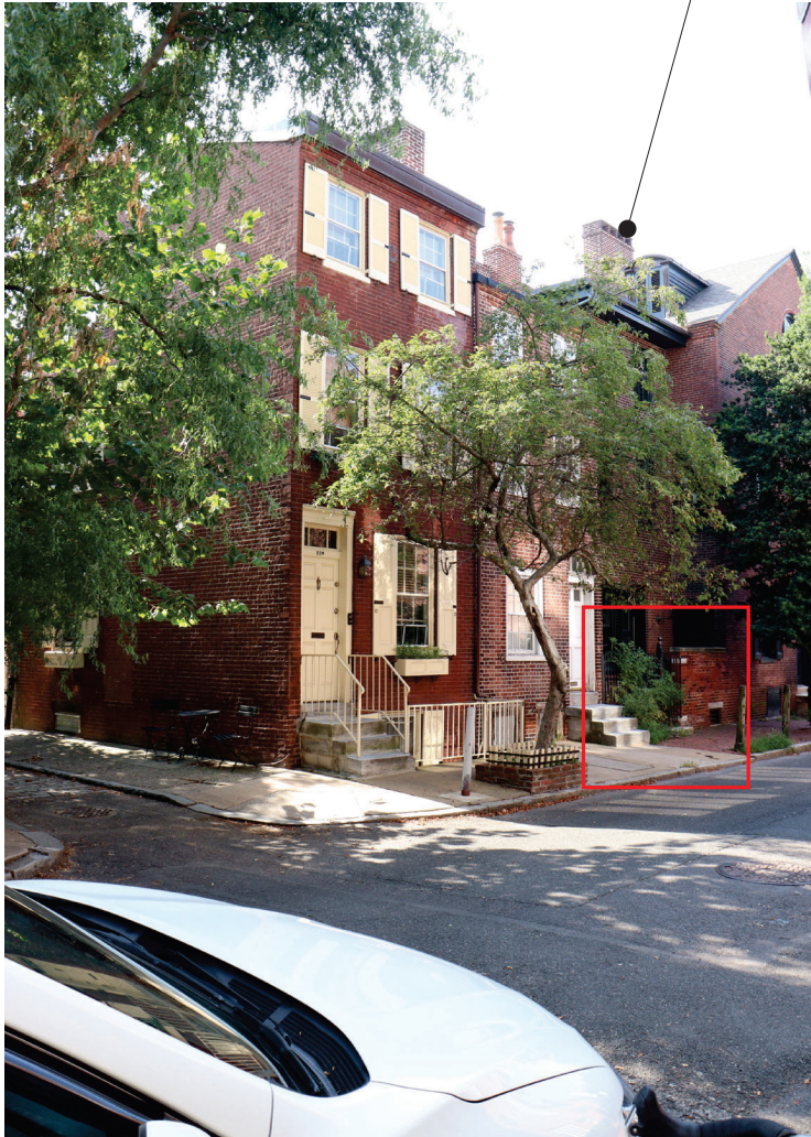
Figure 2: West facade looking down Camac Street, ca. 2025
