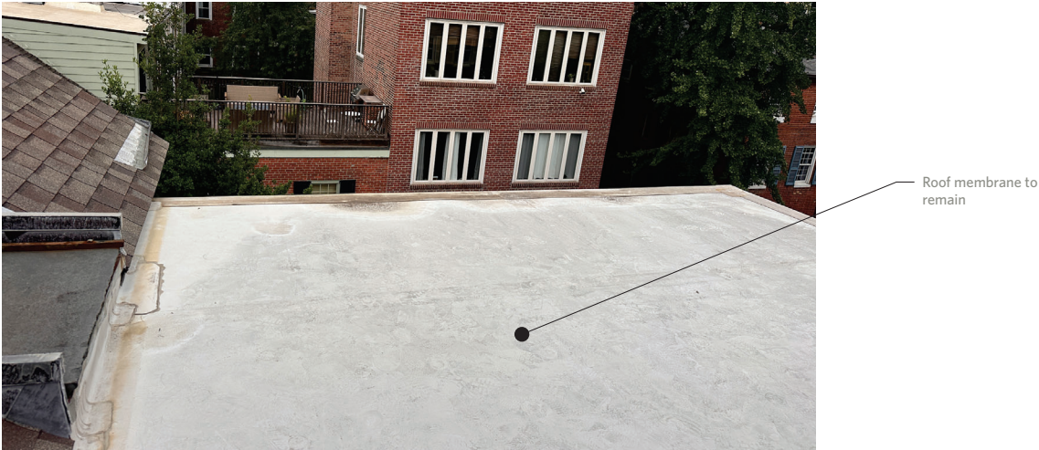
Figure 2: Existing roof membrane
