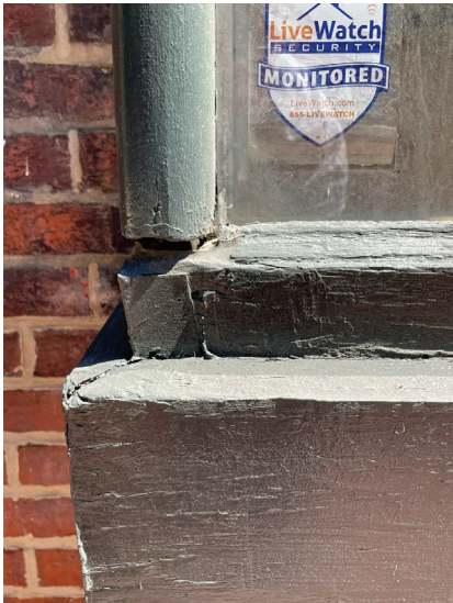
Bay windows show signs of significant structural damage and delamination from the facade. The frames are rotting in places. Single pane glass lights are loose. Both will need to be replaced in kind with painted wood frames and insulated glass.
