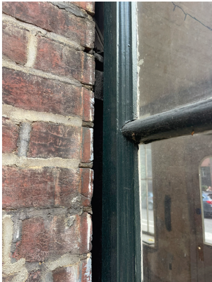
Bay windows show signs of significant structural damage and delamination from the facade. The frames are rotting in places. Single pane glass lights are loose. Both will need to be replaced in kind with painted wood frames and insulated glass.
