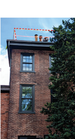
Figure 2: On Camac St, Looking E October 2025
