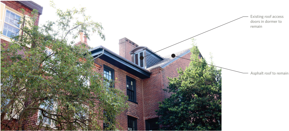
Figure 1: Camac Street view of roof deck
