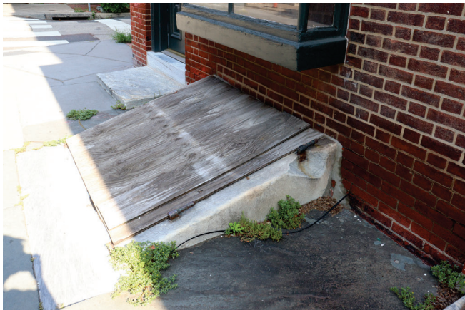
Areaway damage to be repaired, and a new hatch will be added.
