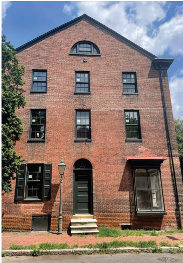
Figure 6: West Elevation, taken from Camac Street July 2025
