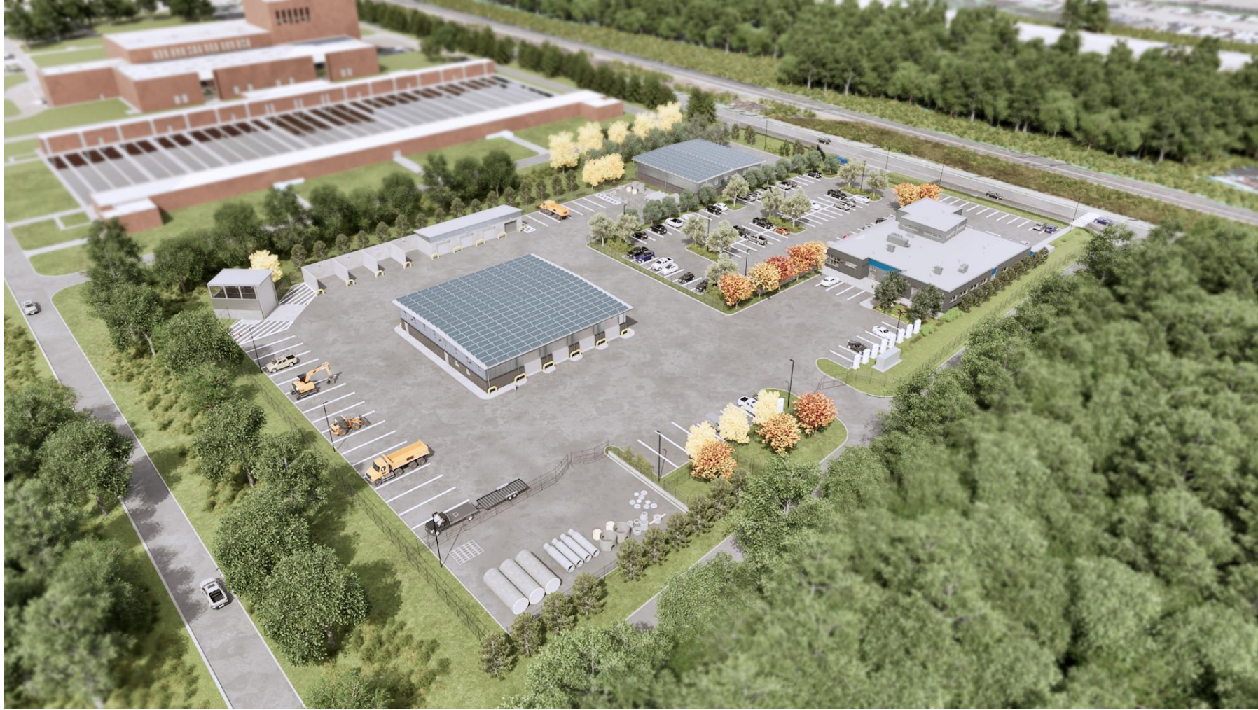
Aerial View from Southwest Corner of Site
