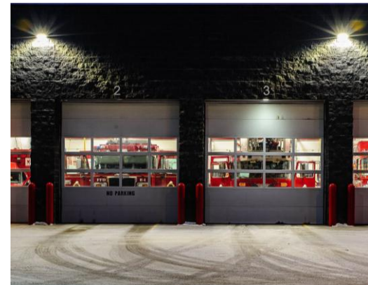
BUILDING-MOUNTED FULL-CUTOFF LED WALL-PACKS
