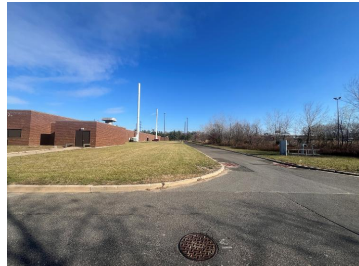
View Looking East From Road G/Road C
