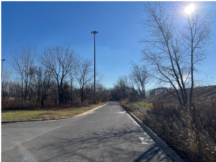
View Looking South From Road G/Road C
