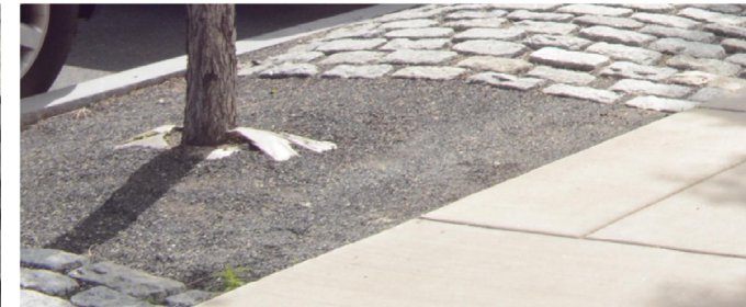
Stabilized stone fines mix at tree opening and polymeric sand in paver joints
