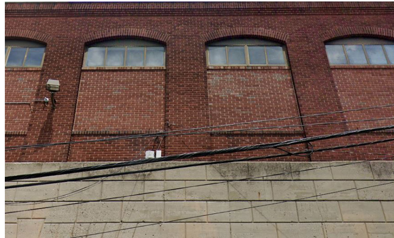
4901 UMBRIA STREET (ON SITE)
