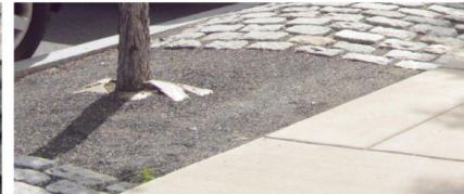
Stabilized stone fines mix at tree opening and polymeric sand in paver joints
