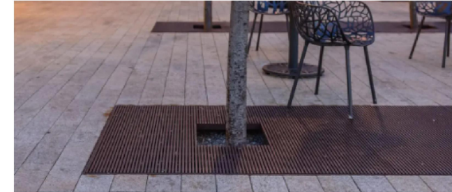
Alternate to street tree pavement below: Urban Accessories, Jamison 3ft x 8ft iron tree grate
