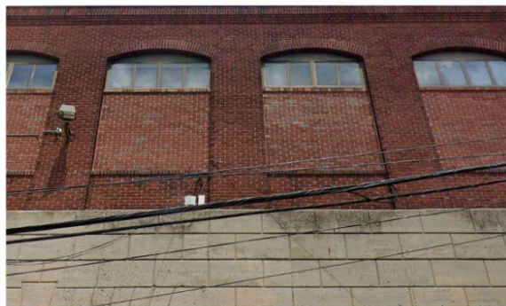
4901 UMBRIA STREET (ON SITE)
