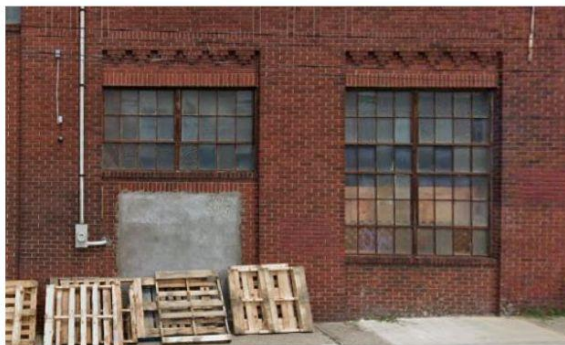
4891 UMBRIA STREET (ON SITE)
