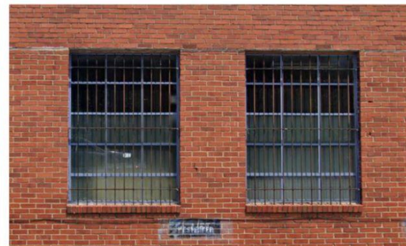
LEMONTE STREET (ON SITE)
