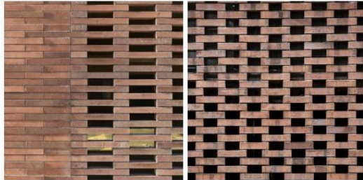
BRICK SCREEN WALL
