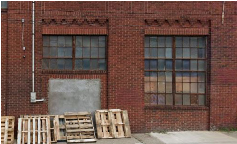
4891 UMBRIA STREET (ON SITE)
