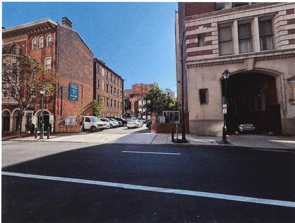
Looking across the street
