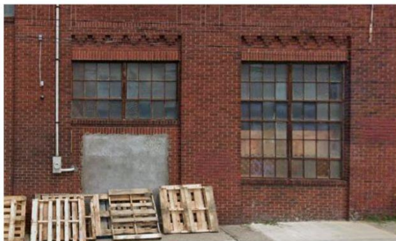
4891 UMBRIA STREET (ON SITE)
