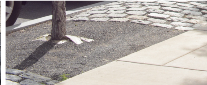
Stone fines mulch at tree opening and in paver joints
