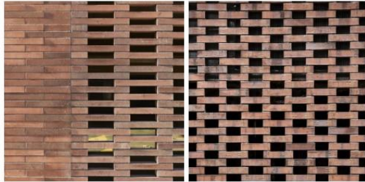
BRICK SCREEN WALL
