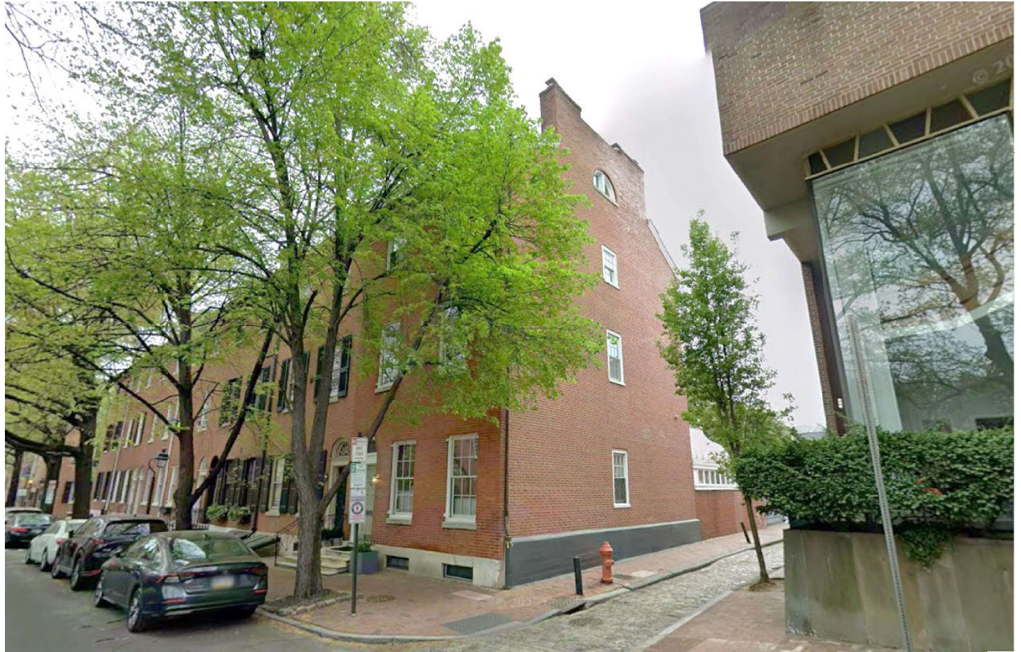
VIEW FROM S 3 RD STREET
