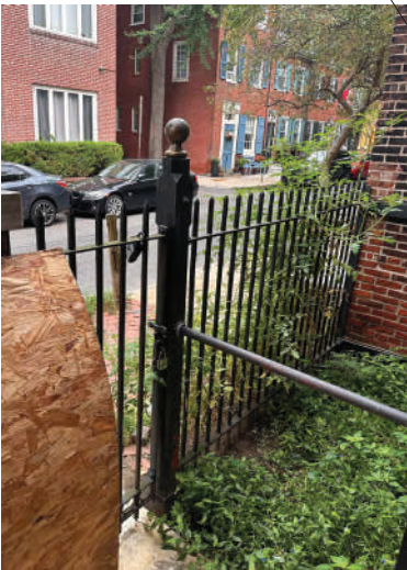
Figure 3: View of metal fence and rail
