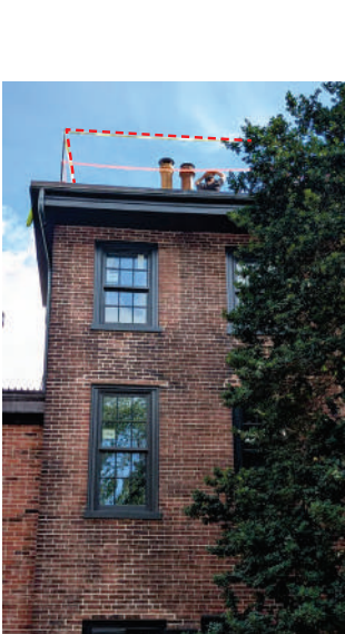
Figure 2: On Camac St, Looking E October 2025
