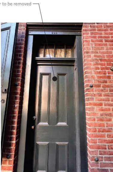
Figure 3: Kitchen entry door
