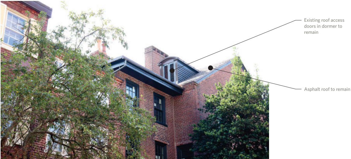
Figure 1: Camac Street view of roof deck
