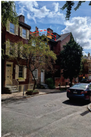
Figure 7: On Camac St, Looking SE October 2025
