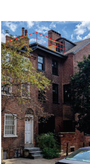
Figure 4: On Camac St, Looking SE October 2025
