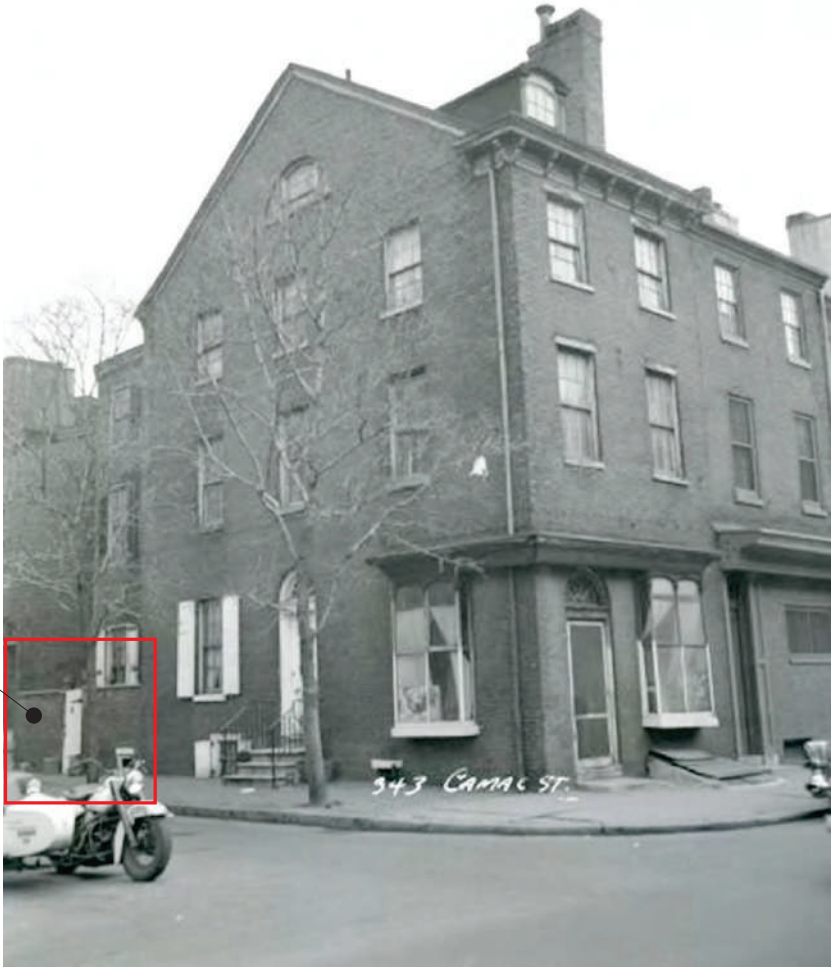
Figure 1: South and West Elevations looking at the intersection of Pine Street and Camac Street, ca. 1959
