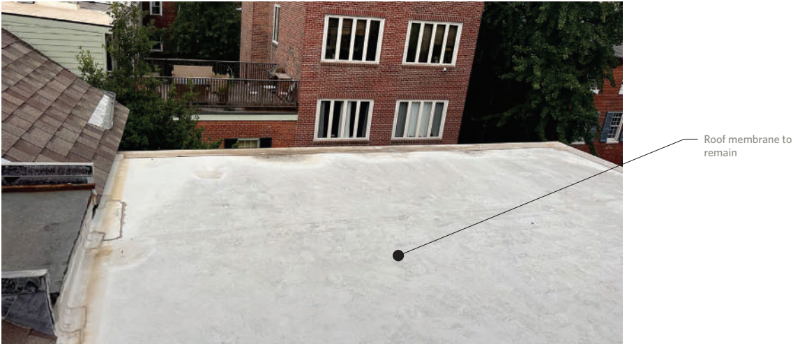
Figure 2: Existing roof membrane
