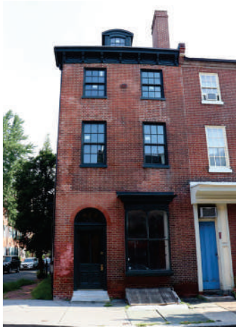
Figure 1: South facade, taken from Pine Street July 2025
