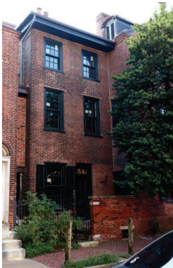
Figure 4: West Elevation, taken from Camac Street July 2025
