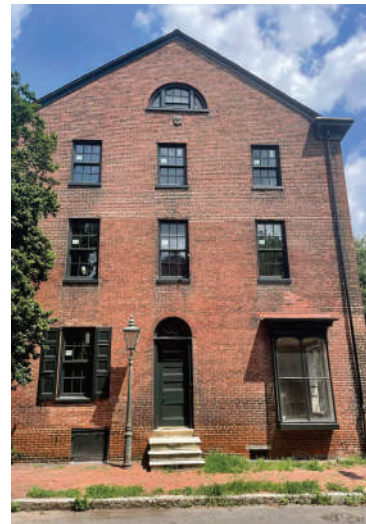
Figure 6: West Elevation, taken from Camac Street July 2025
