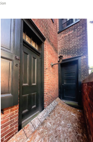
Figure 2: Existing side yard entry doors
