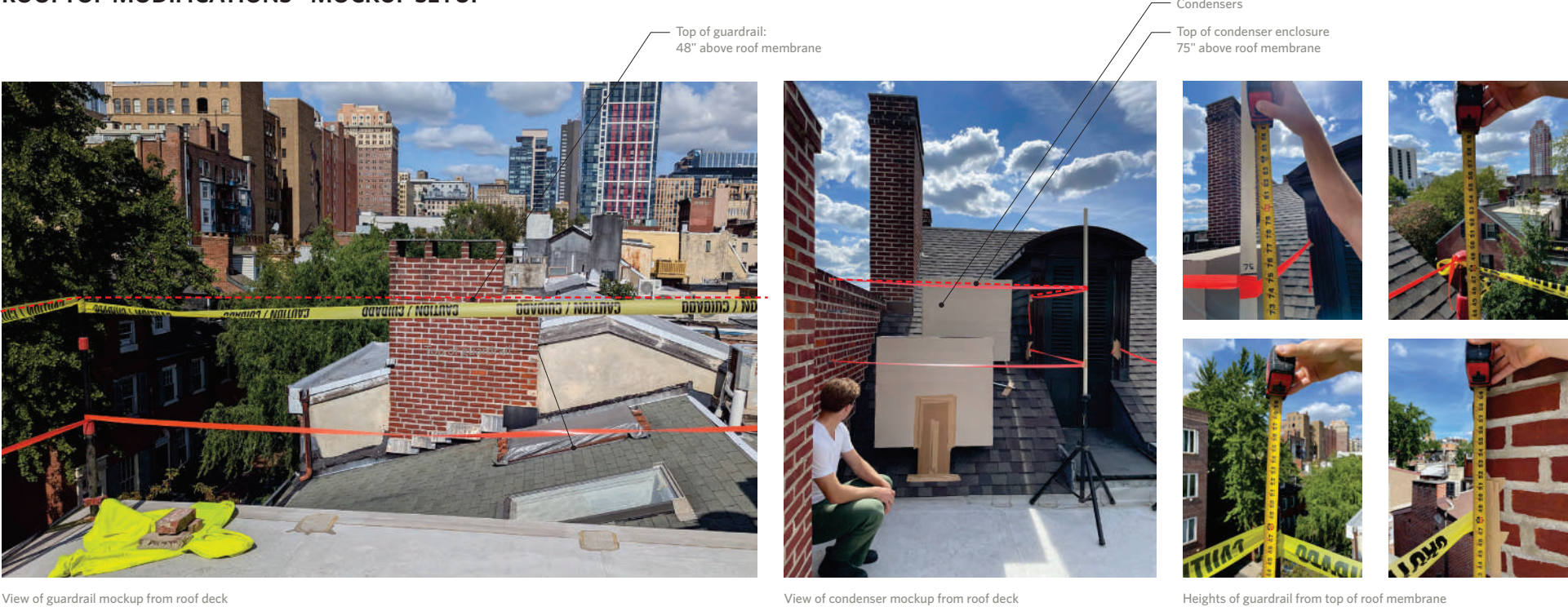
View of guardrail mockup from roof deck
