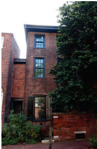
Figure 5: West Elevation taken from Camac Street July 2025
