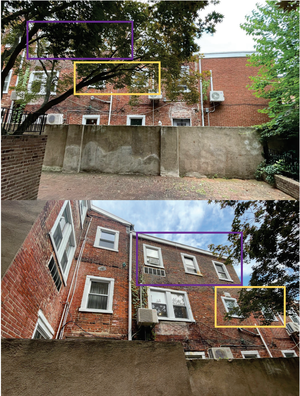
Figure 7: West elevation of 614 Pine St, viewed from the greenway. Window openings in the purple rectangle would be relocated to align with the windows below. Window openings in the yellow rectangle would be lengthened.
