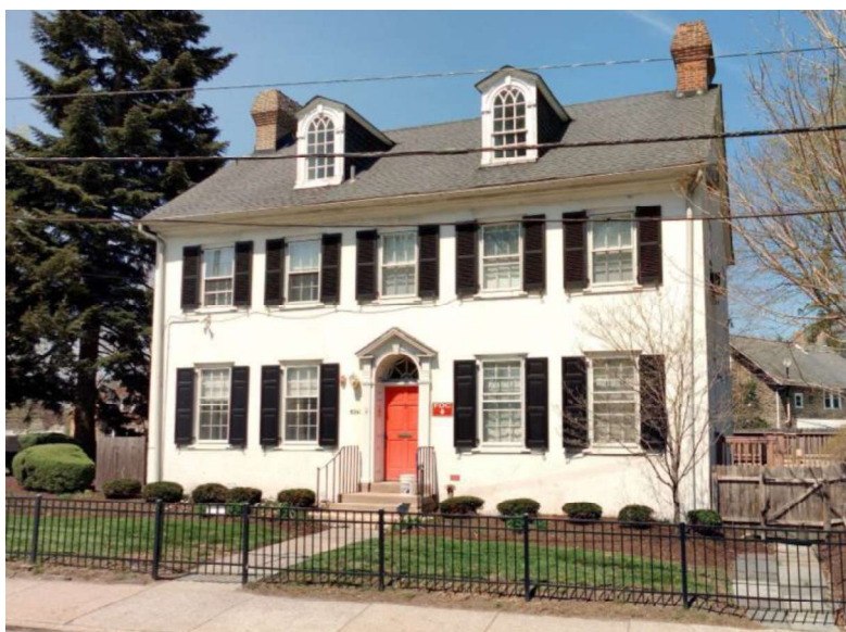
Figure 20. Levering-Jones House, 6341 Ridge Avenue, 1796.
