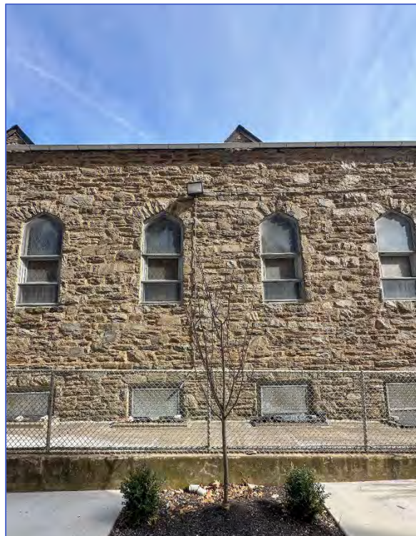
17. Section of west façade. Photo by author.
