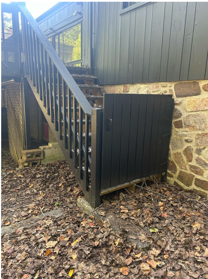
Locked gate to deck.
