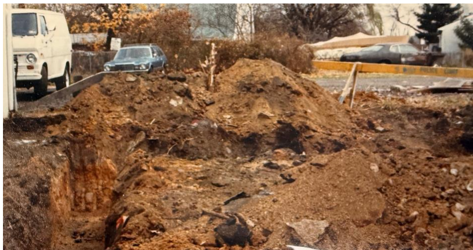
1980s site excavation, looking toward rear of property, site filled for rear paving with clay below
