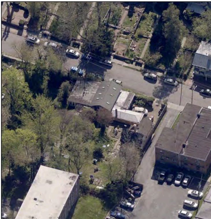
Fig. 3. Aerial photo of 419 W. Clapier Street from the southwest. Source: Pictometry, the Office of Property Assessment, City of Philadelphia. Accessed March 29, 2025.
