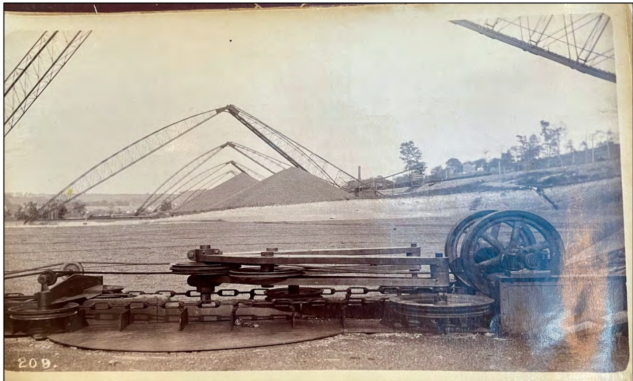
Fig. 76. An undated photo of Jamie Dodge's innovative coal storage mechanism with coal piles in the background. Source: Donald and Robert M. Dodge Collection, Firestone Library, Princeton University.
