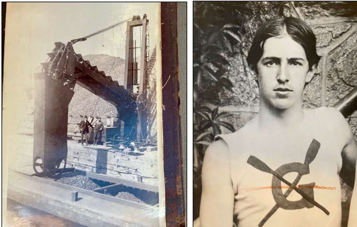
Fig. 77, left. An undated photo of James Mapes Dodge's coal storage invention showing how the mechanism can load from piles into transport containers as well as in reverse to load the piles. Source: Donald and Robert M. Dodge Collection, Princeton. Fig. 78, right. An 1898 photo of son Kern Dodge at Germantown Academy. Source: Philadelphia Record Photo Morgue, Historical Society of Pennsylvania.
