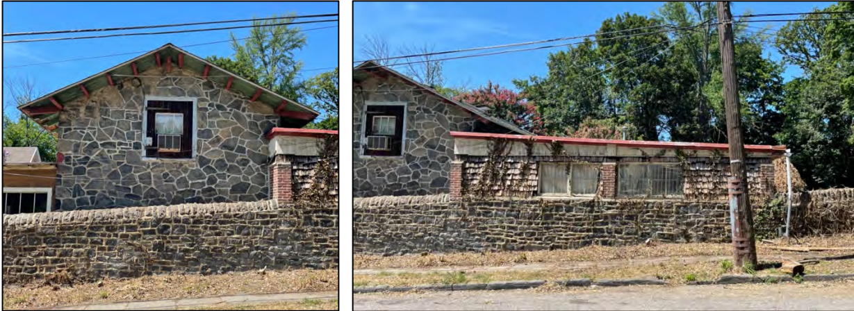
Fig. 19, left. The east elevation of the stone building between the garage to the south and the solarium to the north. Fig. 20, right. The east elevation of the solarium to the north of the stone building. The shingled panels are not original; they cover windows. The east perimeter wall is the base of the east solarium wall. Photos dated August 9, 2025.
