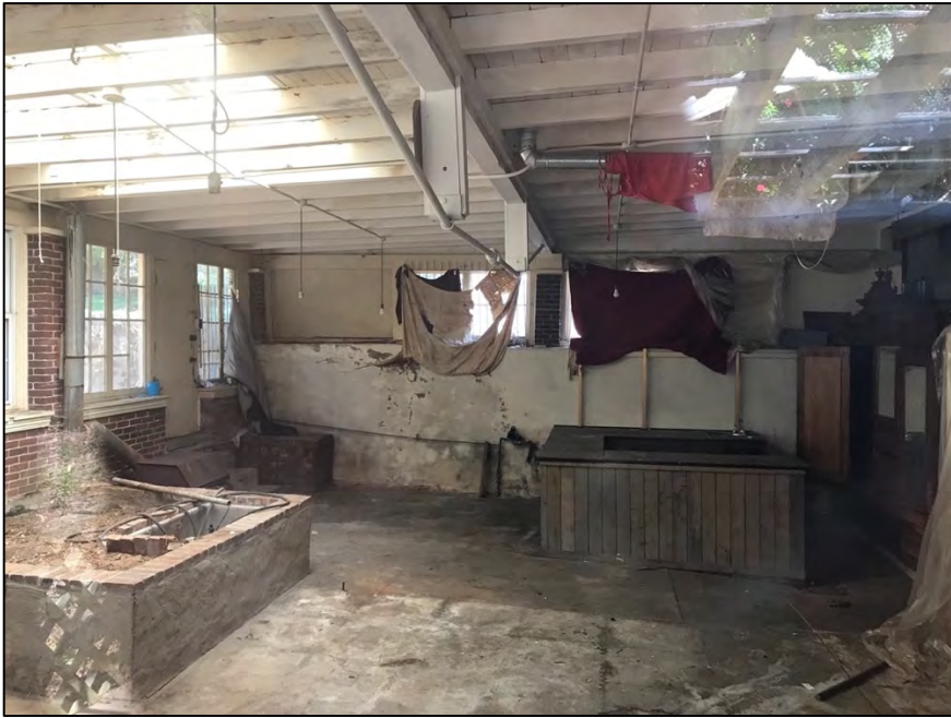
Fig. 25. The interior of the solarium from the garden-facing windows. There are skylights at the northern side of the roof (right side; left side shows reflection of the exterior pergola structure) and below it what seems to be a piped structure. There are exposed concrete floors and rafters. The east side (opposite) shows the windows on each far end boarded up by plywood (and faced at the exterior by shingles). There is a parge coat on the interior side of the east perimeter schist wall with a more structured sill. Date: August 11, 2025.
