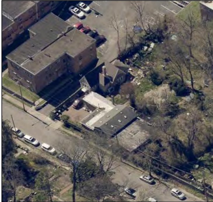
Fig. 2. Aerial photo of 419 W. Clapier Street from the northwest. Source: Pictometry, the Office of Property Assessment, City of Philadelphia. Accessed March 29, 2025.
