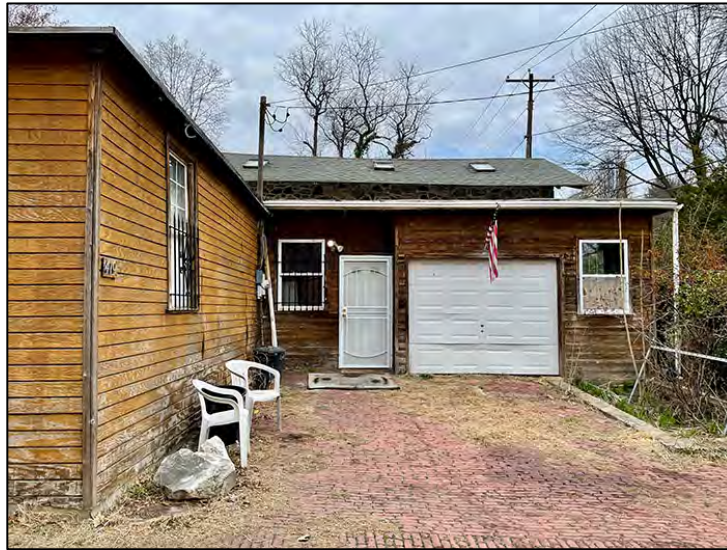
Fig. 12. The garage with L-shaped footprint wrapping the motor court. The roof of the earlier stone building containing three skylights is beyond. Date: March 28, 2025.
