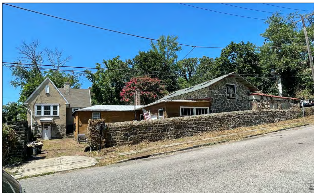
Fig. 6. A view of the subject property along Clapier Street with the motor court in front of the 1923 cottage to the left, the garage, a stone building, and a solarium. There is a schist perimeter wall at the south and along the street that terminates at McKean Avenue, underscoring the once unified parcels of 5000 McKean. There is photographic evidence that the wall was constructed after the 1910 solarium was built and that the perimeter was enclosed previously by a metal hairpin fence which was used throughout the neighborhood in the late nineteenth century. Date: August 9, 2025.
