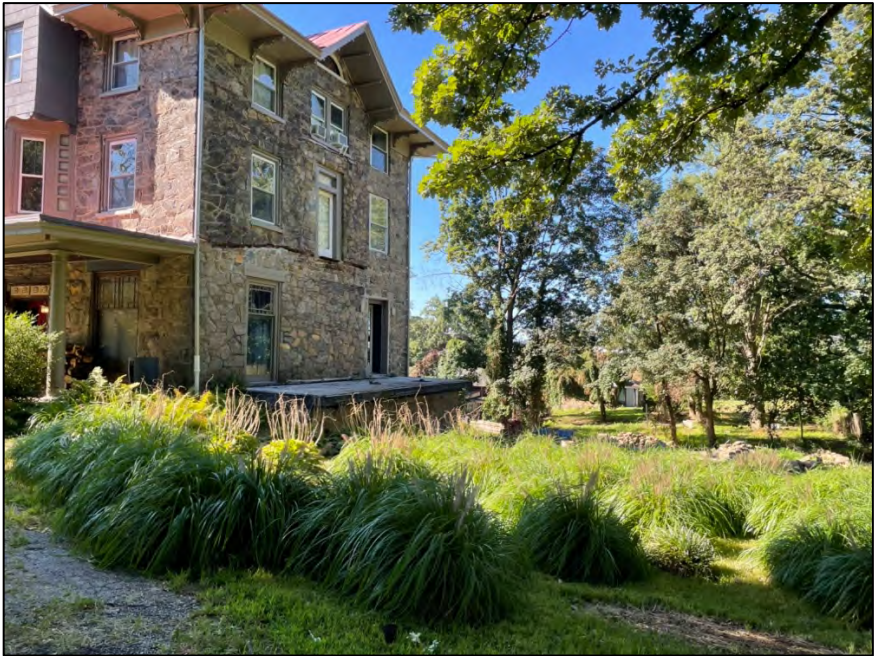
Fig. 48. View from the governor's driveway at 5000 McKean Avenue looking down the rear yard into the subject property. The rear door to the Cottage can be seen in the middle distance. Date: August 26, 2025.
