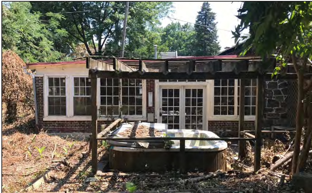
Fig. 24. The west elevation of the solarium faces the garden and a pergola structure under which currently is a hot tub. There are double doors between a slate patio and the interior. Date: August 11, 2025.
