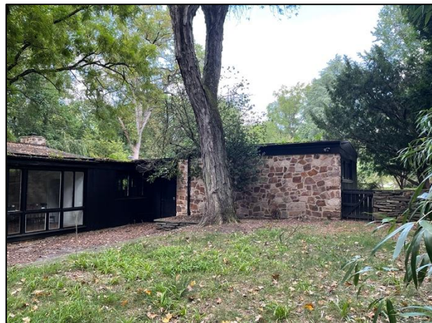
Figs. 18 & 19. The west elevation of the staff quarters wing is clad entirely in Valley Forge stone except for a door near the kitchen accessible from a private patio. Date: August 29, 2025.
