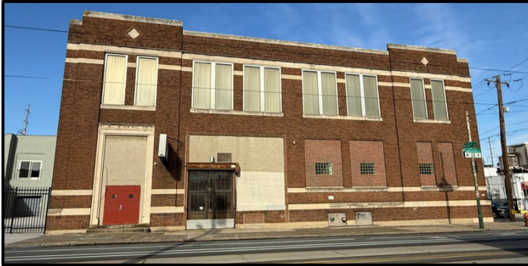
Figure 5. The primary (south) elevation. Source: Oscar Beisert, 2025.
