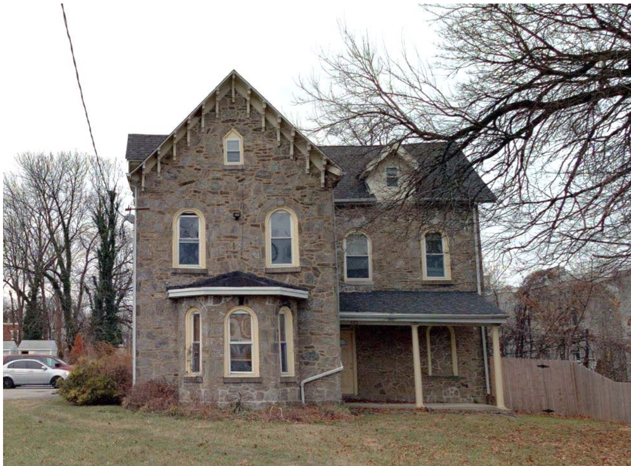
Figure 1: Photo of subject property at 723 Church Lane from Cyclomedia.
