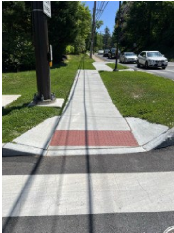
ADA curb ramp in the forefront, with a grass area as crossing ban treatment to the right of the curb ramp.
