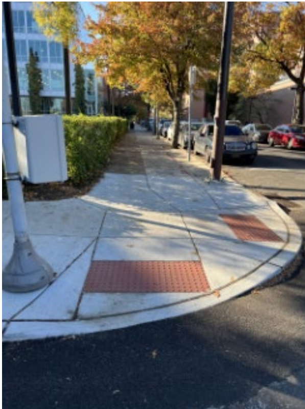
ADA Curb Ramps at various locations
