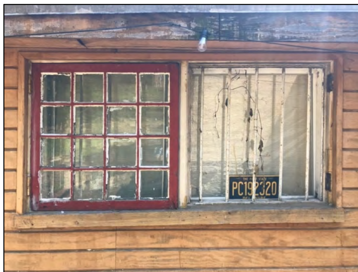
Fig. 14, left. The junction of the north elevation of the stone building and the garage's workshop extension. Date: July 27, 2025. Fig. 15, right, the southernmost window opening in the west elevation of the garage's workshop extension showing what may be an original cased wood window with divided lites. Date: August 9, 2025.
