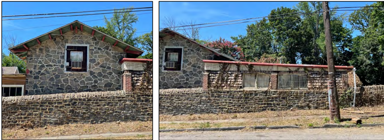
Fig. 18, left. The east elevation of the stone building between the garage to the south and the solarium to the north. Fig. 19, right. The east elevation of the solarium to the north of the stone building. The shingled panels are not original; they cover windows. The east perimeter wall is the base of the east solarium wall. Photos dated August 9, 2025.
