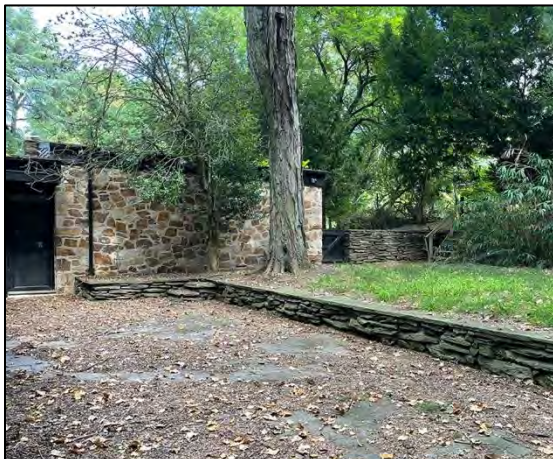
Figs. 18 & 19. The west elevation of the staff quarters wing is clad entirely in Valley Forge stone except for a door near the kitchen accessible from a private patio. Date: August 29, 2025.
