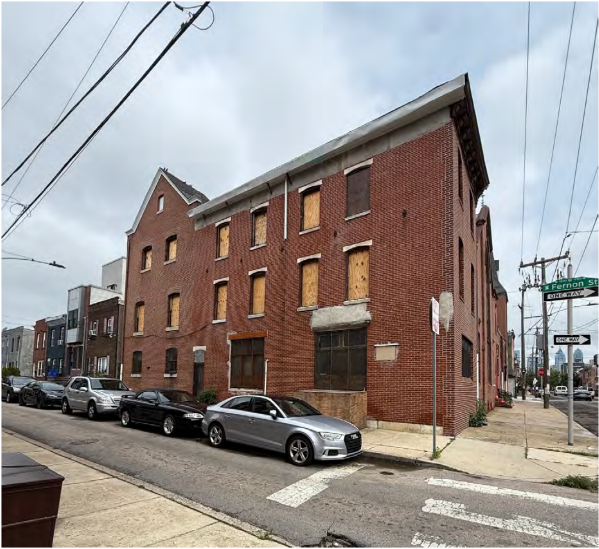
Fernon Street façade
