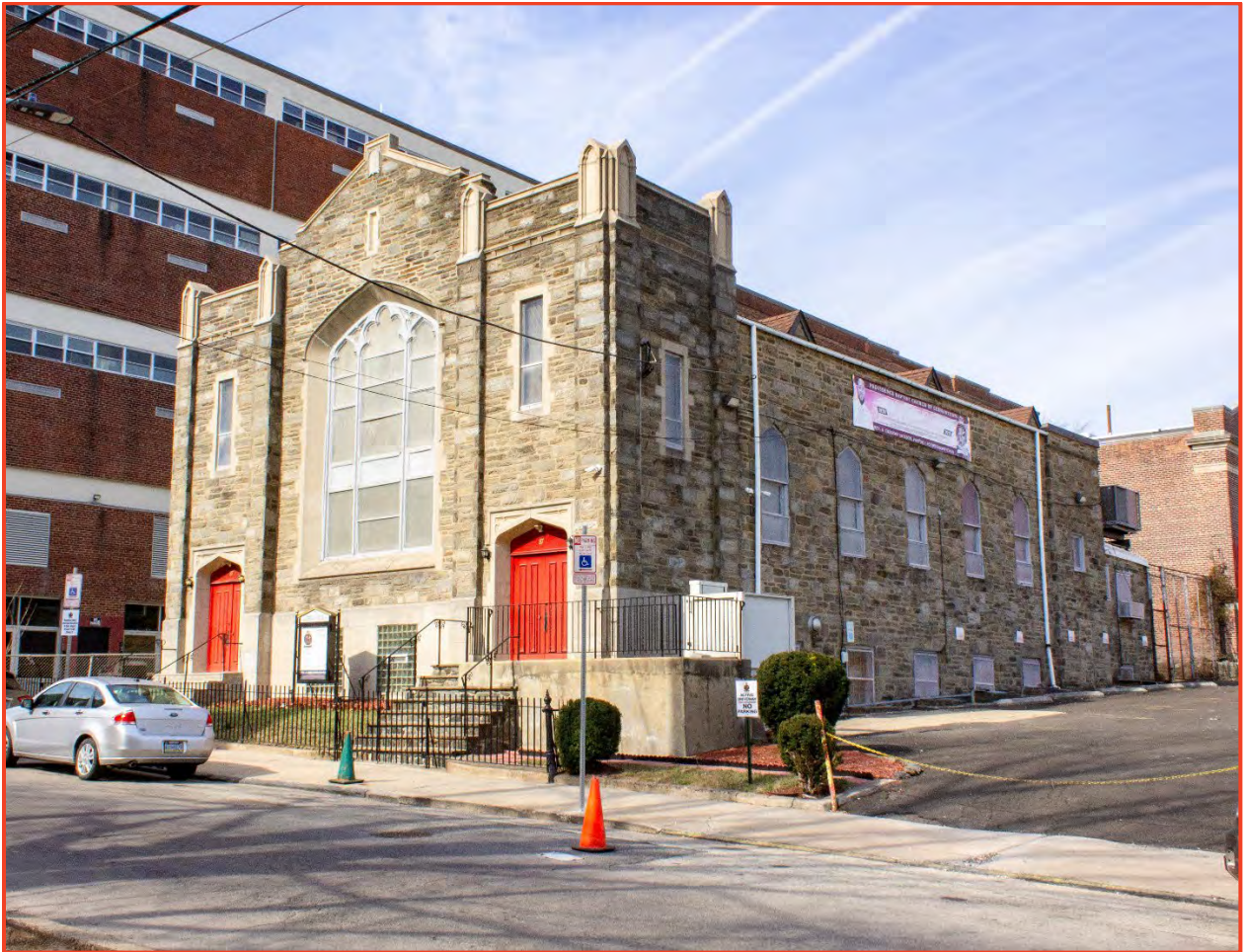
Providence Baptist Church built 1940-1943
