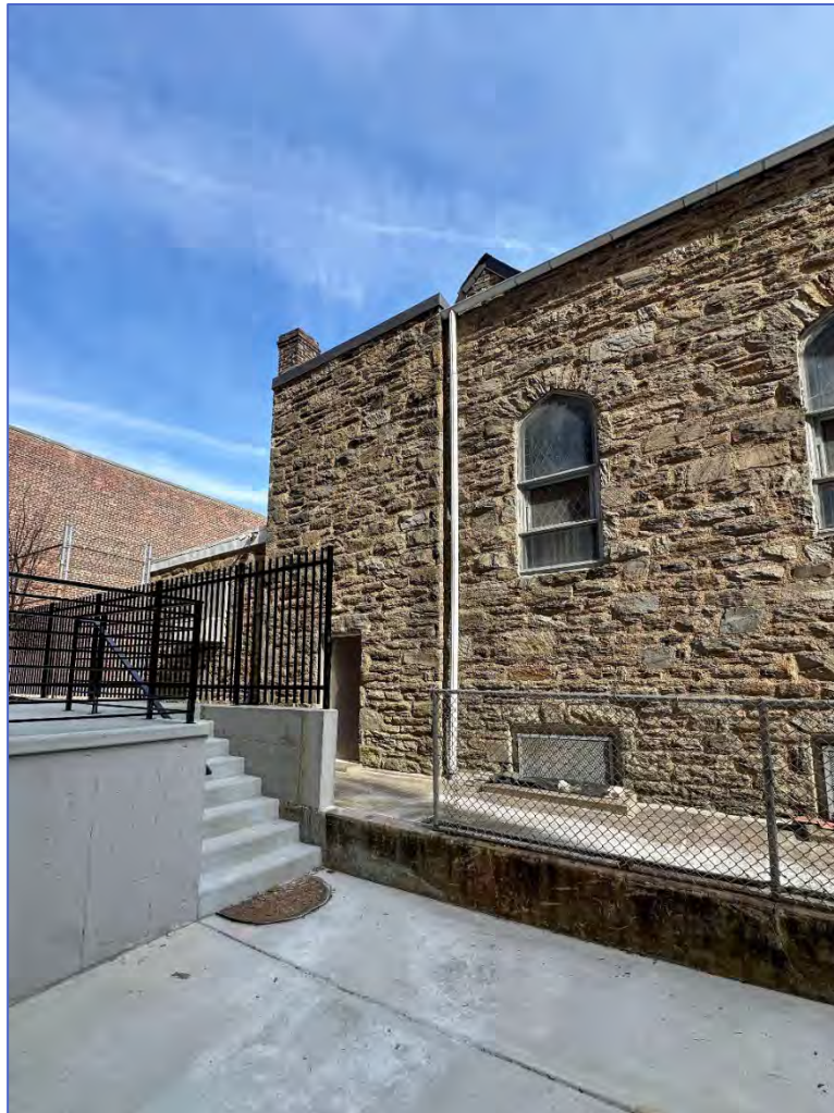
18. Rear of west façade. Photo by author.
