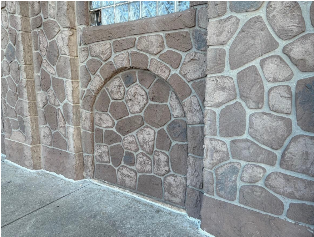
Image 9: Close up view of stone veneer along N. 17 th Street.
