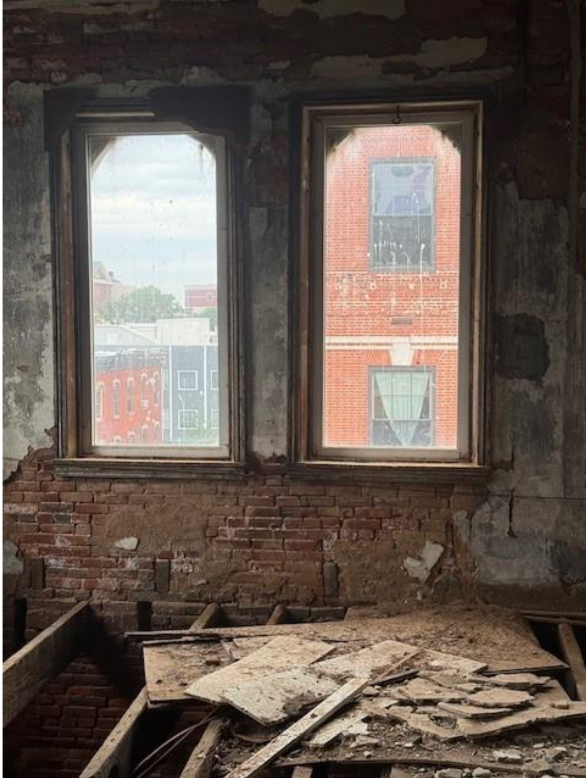
Image 11: Interior view of windows on third floor. Plaster was removed to expose original brick. There is no indication that these windows were reduced in height since the 1859 construction. The lack of alterations in this area confirms that the brick panel detailing on the exterior was included in the original design and construction.
