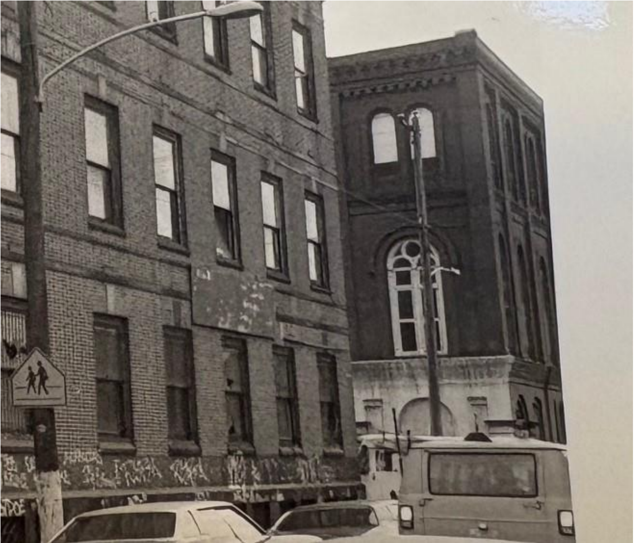
Image 12: 1632 Poplar Street in early 1980s. Photograph shows building corner at Poplar and N. 17 th Streets. Unpainted brick is visible on the second and third levels. The first floor appears to have stucco applied to the façade and window/door openings are filled in. An original window is still visible on the second-floor façade. The architectural design of Philadelphia public markets constructed during the mid-18 th century consistently showcased heavy ornamented brick and large arched windows with detailed tracery. The original window shown in this photo is similar to other public markets constructed in this era (see Images 13-16) .
