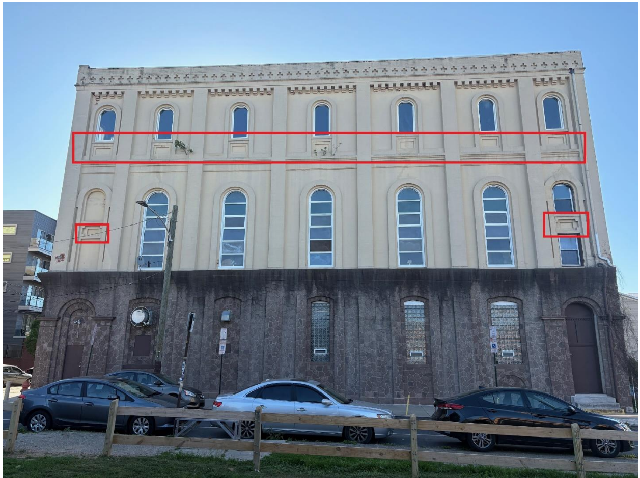
Image 10: Elevation along N. 17 th Street. The red boxes show areas of historic brick detailing that dates to original construction. The third floor recessed panels are also extant on the Poplar Street front façade.
