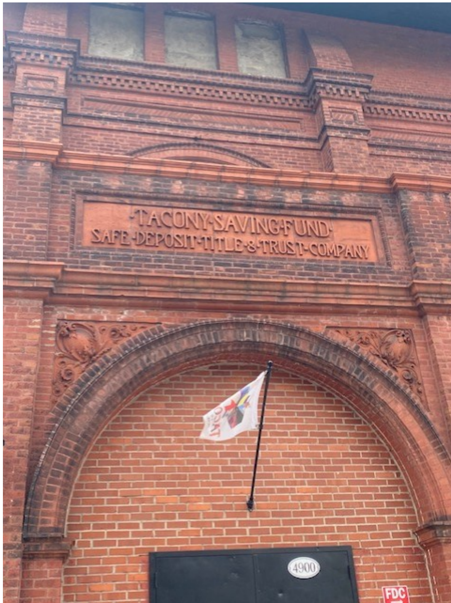
Figure 23. Tacony Saving Fund Safe Deposit, Title & Trust Co. terra cotta and brick primary facade detail.
