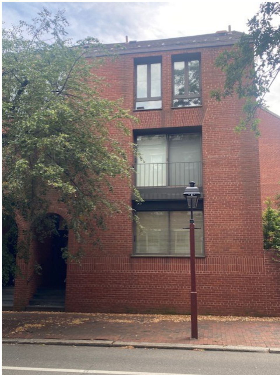
Figure 3. 310 Spruce St. front (north) facade
