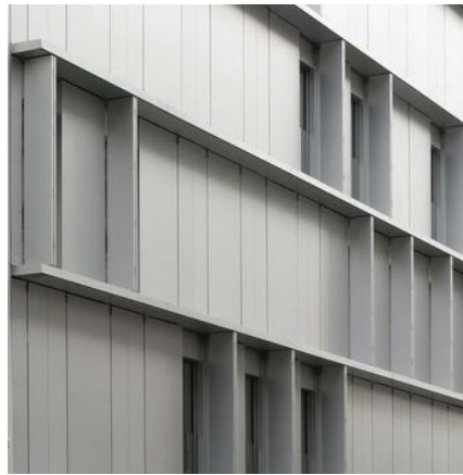
4 METAL PANEL ALUMINUM COMPOSITE PANEL WITH SMOOTH FINISH COLORS AS SHOWN IN ELEVATIONS
