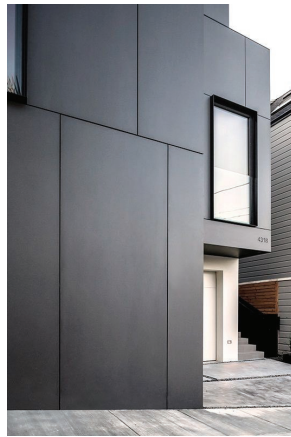
4 METAL PANEL ALUMINUM COMPOSITE PANEL WITH SMOOTH FINISH COLORS AS SHOWN IN ELEVATIONS
