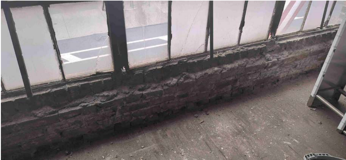
Photo 4 – front wall is bowing out and masonry is deteriorated
