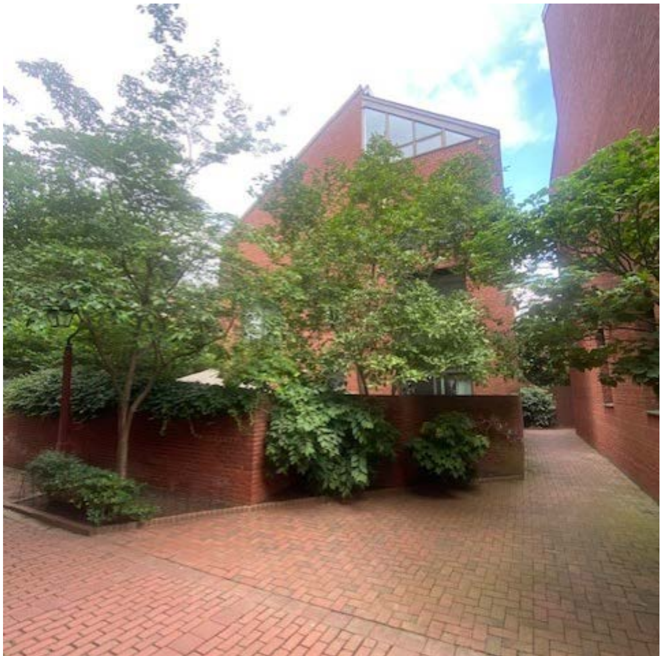
Figure 4.310 Spruce Street west facade
