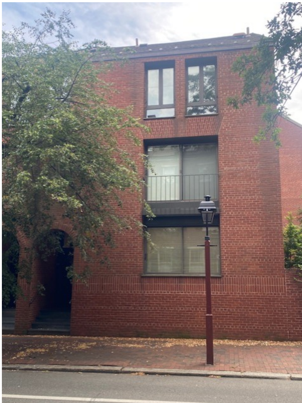
Figure 3. 310 Spruce St. front (north) facade
