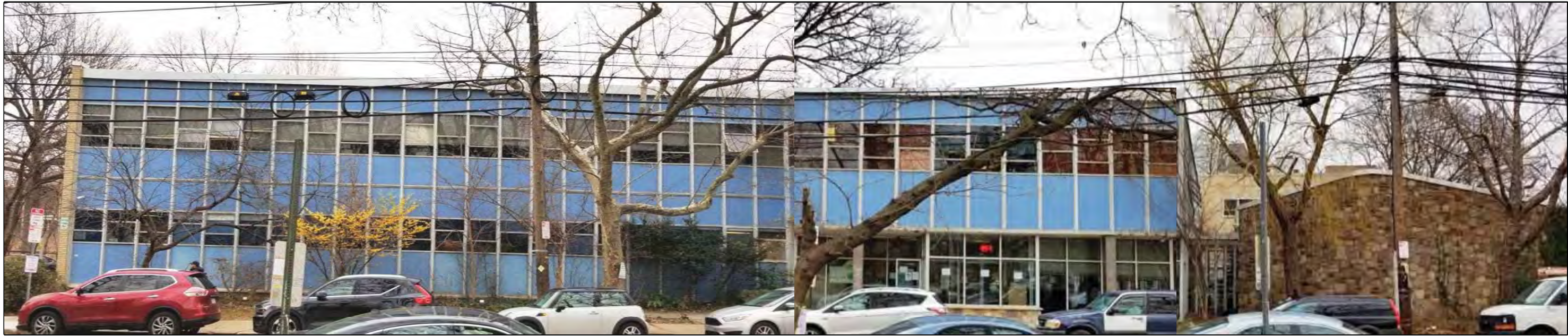
1) Health Care Center No. 3 Front Elevation with Entrance Facing Clark Park across 43rd Street
