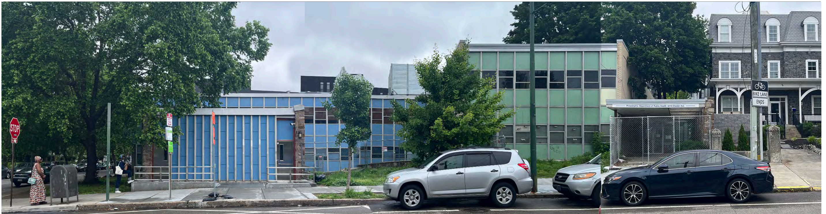
1) Chester Avenue Elevation, south side of building with Vacant Phipps Wing and Entrance Canopy on uphill East Side (Right Side of Photo)
