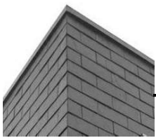
Synthetic or Natural Slate tiled façade @Penthouse level
