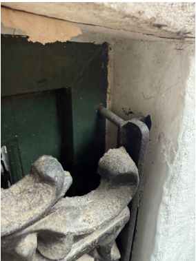
EXISTING WINDOW GATE CONNECTION
