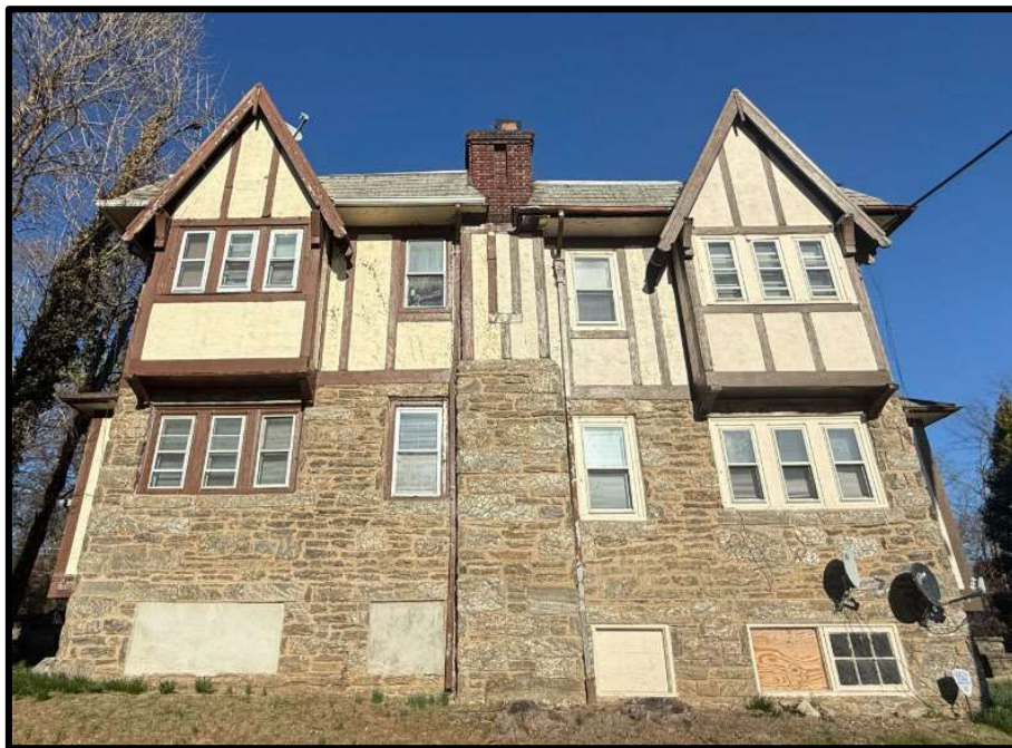
Figure 29. The southwest elevations of 6605 (on right) and 6607 (on left) Blakemore, showing the more typical vertical half timbering. Source: Oscar Beisert, 2025.
