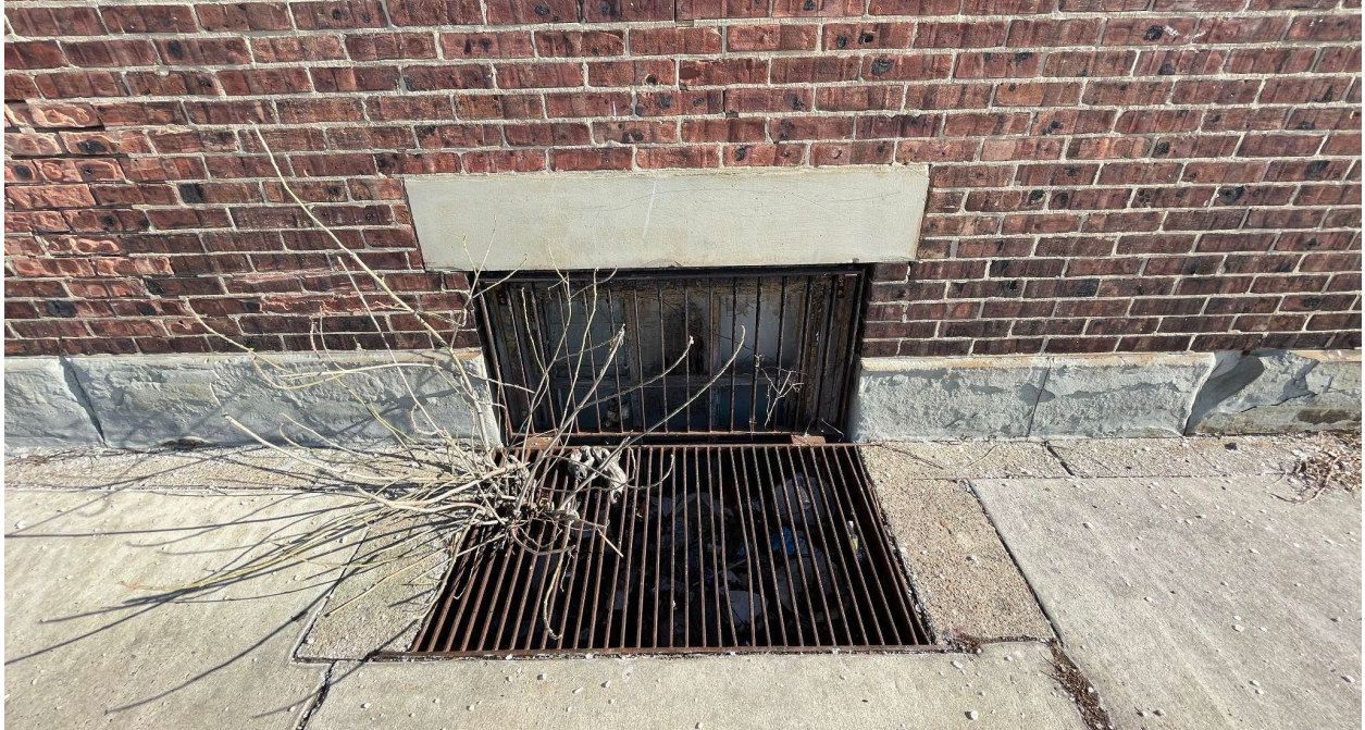
FIGURE 9: West elevation basement light well showing bluestone lintel and an original window. (PC)
