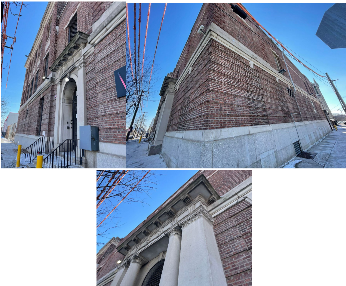
FIGURE 13: Verizon building (formerly Bell Telephone), southwest corner of Lancaster and Bible. Note stylized Flemish bond, entablatures, and keystones. (Joseph E. DeStefano, January 2025)
