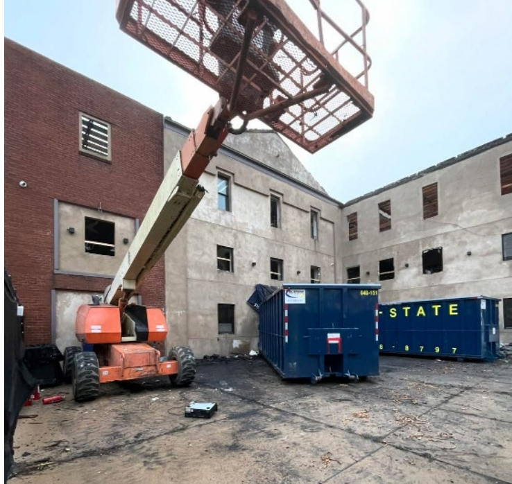
FIGURE 17.1: The first location of the George Institute at 5100 Lancaster Avenue being demolished on March 5th, 2024. The central portion dates to the library’s 1872 opening and retained its basic historic form. This vernacular, almost Greek Revival, structure featured a front gable, square pilasters at each corner, and a dropped cornice that blends into an exaggerated front-spanning lintel. This hefty, front-spanning element gives the upper windows a “hooded” look. (Joseph E. DeStefano)
