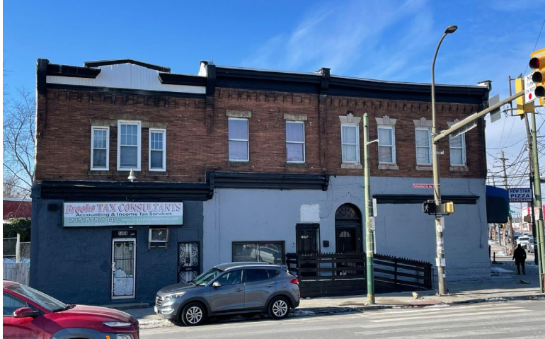
FIGURE 12: Similarly aged row on the southwest corner of 52nd and Lancaster. Note splayed lintels and keystones along with fanlight transom over the door. (Joseph E. DeStefano, January 2025)
