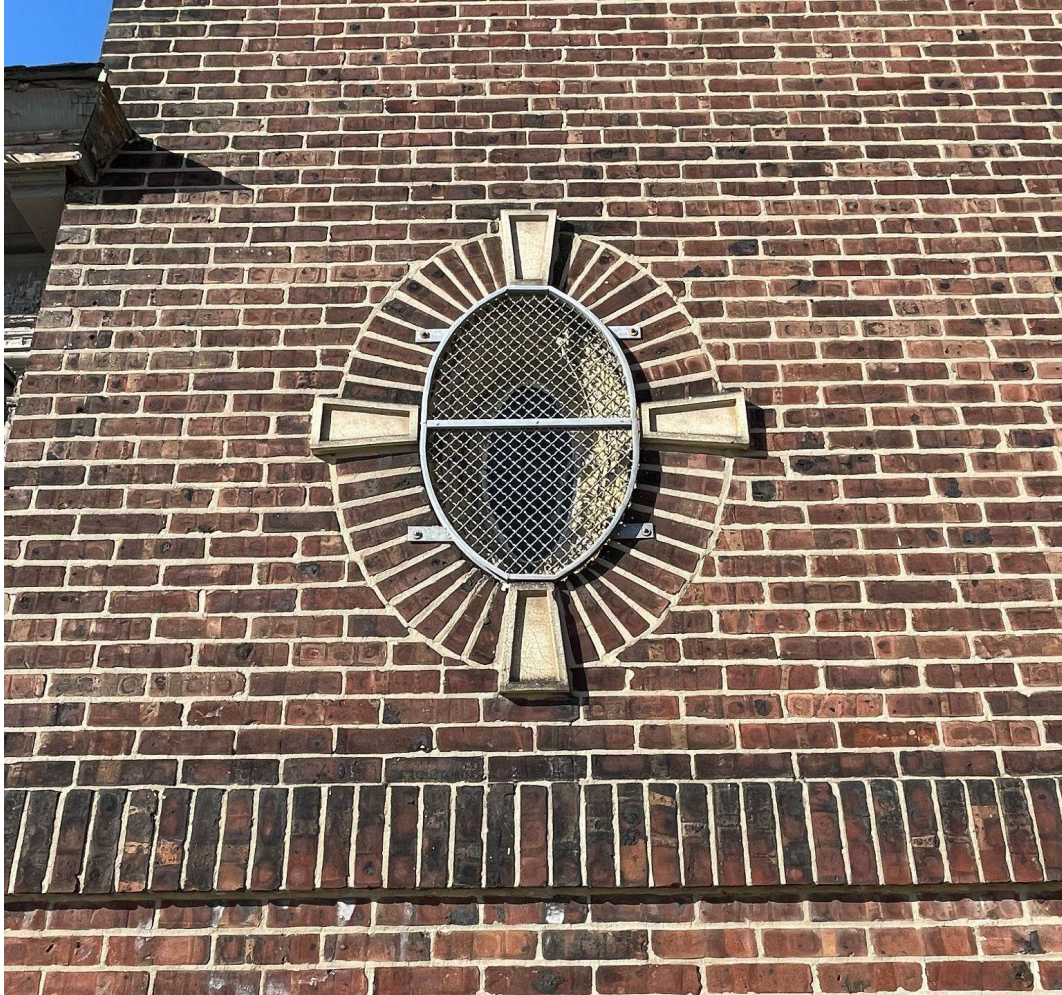
FIGURE 5: First level elliptical windows found towards the southern end of the building on the east and west elevations. Soldier course band in view beneath window. (PC)
