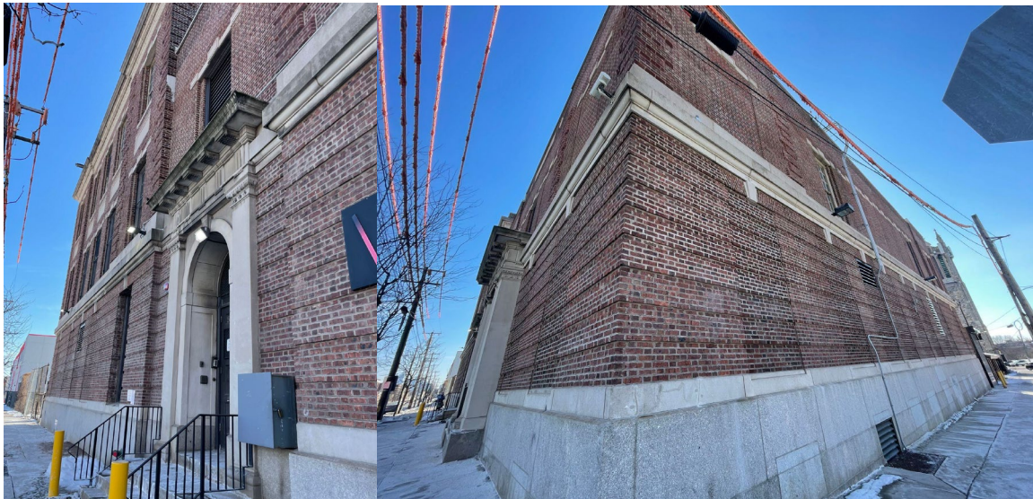
FIGURE 25.1: Restated for reference. Verizon building (formerly Bell Telephone), southwest corner of Lancaster and Bible. Note classical features tied to Federal Revivalism, including stylized Flemish bond, entablatures, and keystone. (Joseph E. DeStefano, January 2025)
