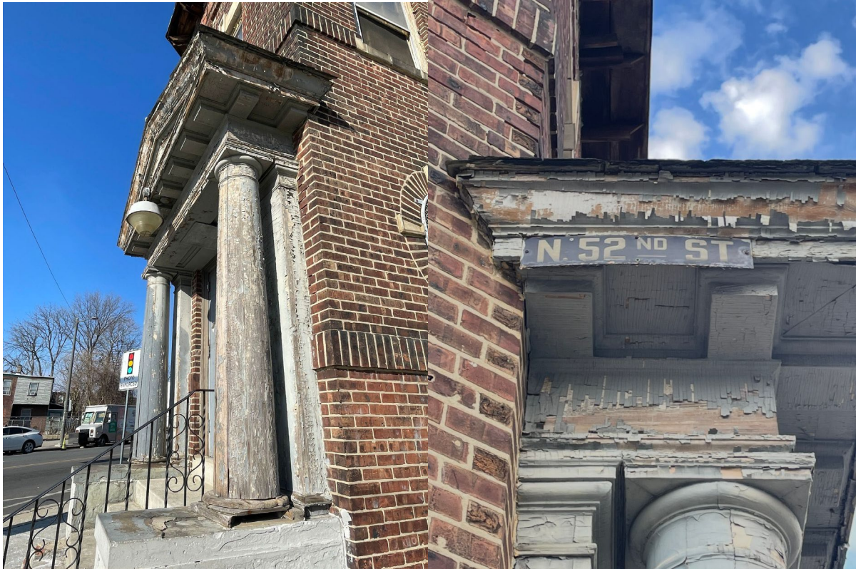
FIGURE 3 + 3.1: Close-ups of the south elevation entrance, showing Tuscan columns, pilasters, modillions on classical entablature/pediment. The right-hand picture (3.1) displays the porcelain enamel street sign. (PC)
