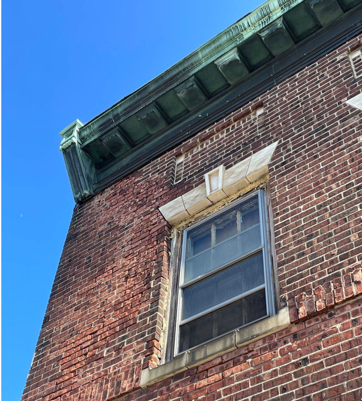
FIGURE 8: Top left corner of west elevation, featuring a portion of intact copper cornice, bracketed cornice end cap, and typical (periphery) rectangular window with splayed lintel, relief-carved keystone, and multi-part sill. (PC)
