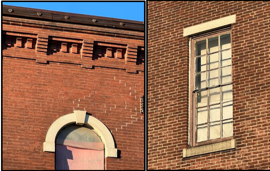
Figure 6a. Left: Window header and cornice detail, Primary (South) Elevation. Figure 6b. Right: An original window, Side (West) Elevation. Source: Oscar Beisert, 2024.
